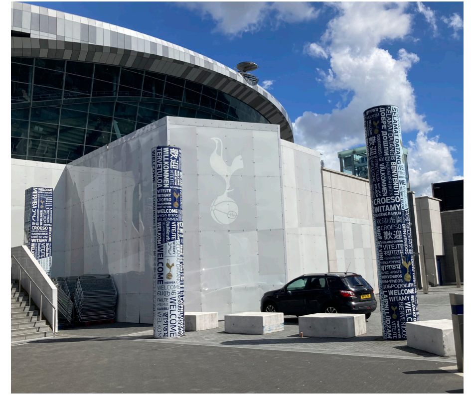
Fig. 3.7: Park Lane. Plot 3 is seen in the foreground and the Stadium (Plot 1) in the background.
