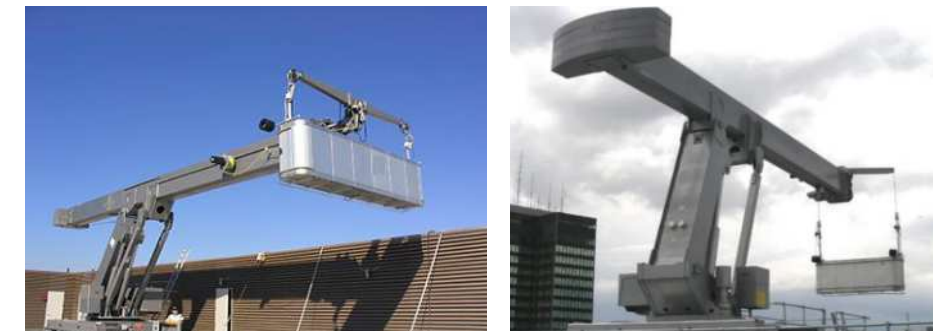
FIGURE 312. Proposed BMU unit equipped with telescopic jib
