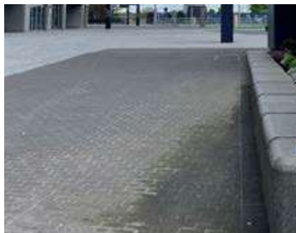
Existing paving at podium level
