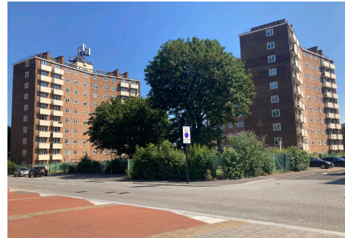
Fig. 6.6: The Charles and Moselle Houses, part of the Love Lane Estate seen from the White Hart Lane Station square.
