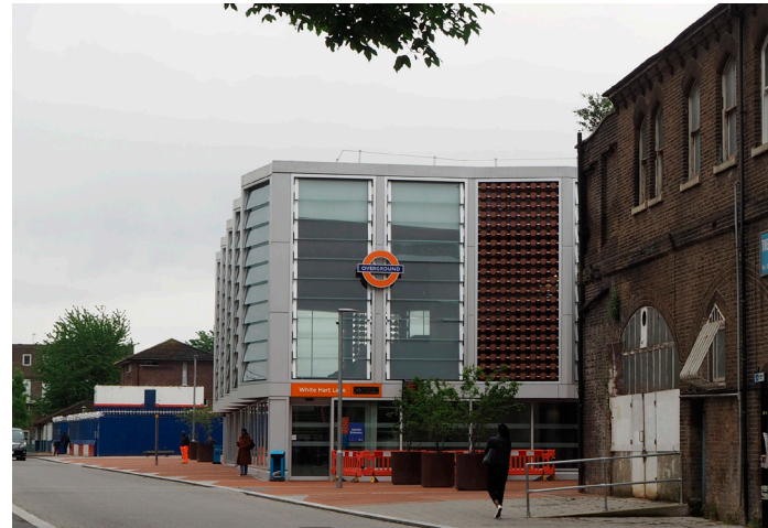
Fig. 6.5: White Hart Lane Overground Station.
