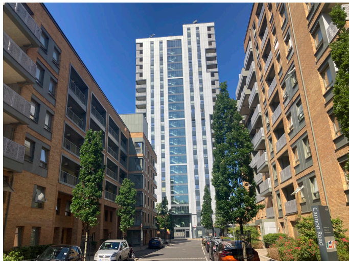
Fig. 6.8: The 23-storey Rivers Apartment, seen from Cannon Road, west of the High Road.
