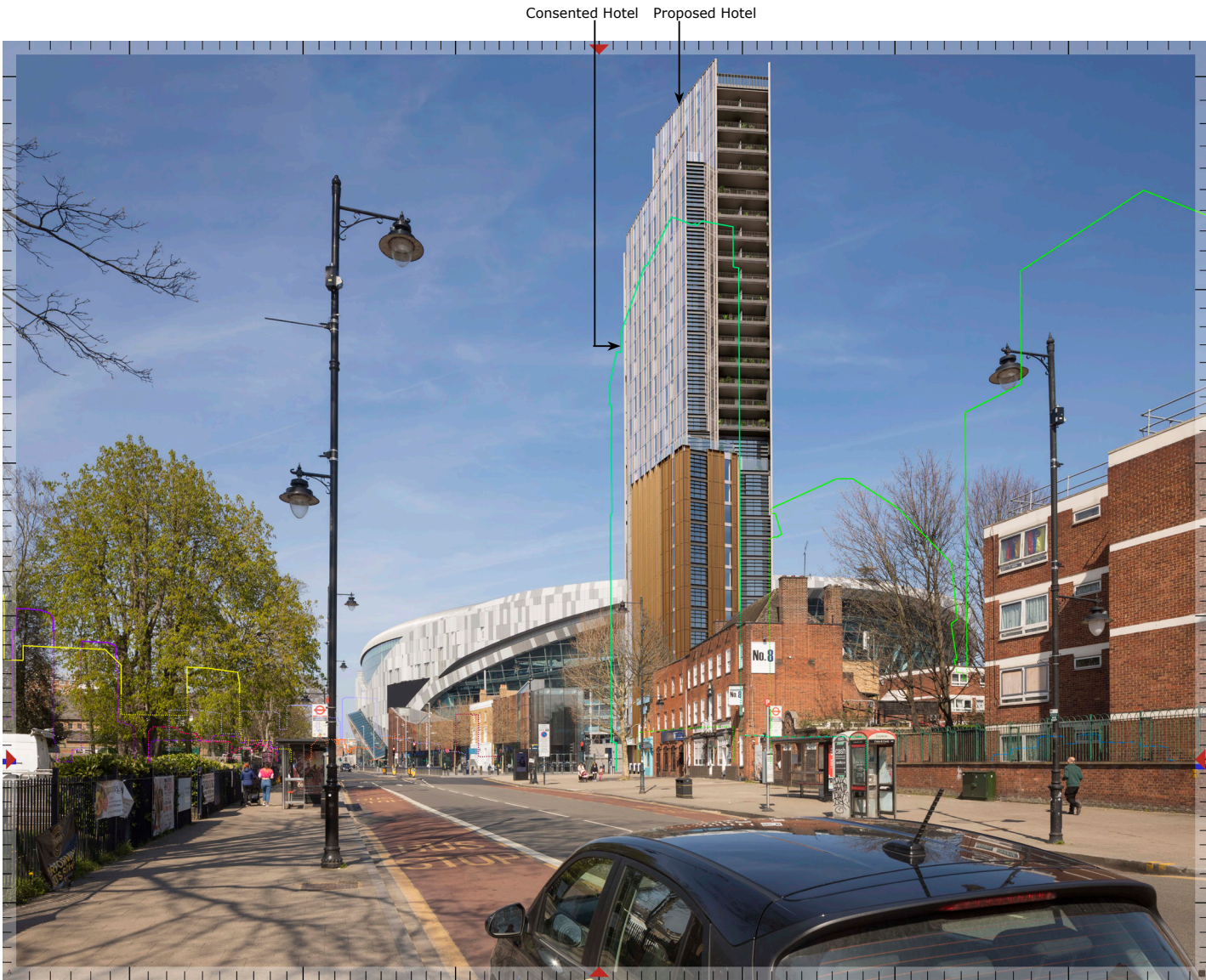
VIEW 22 - HIGH ROAD AT BROMLEY ROAD
