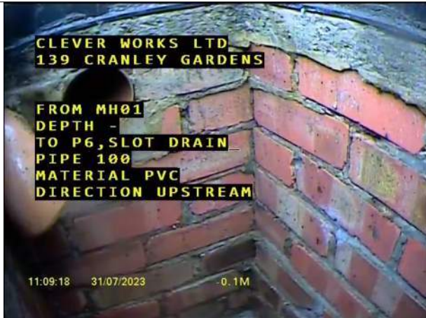
00:00:00, 0.00 m Start manhole, MH01
