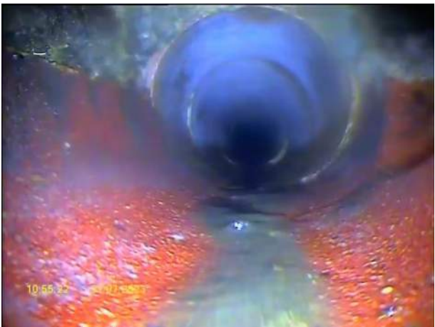
00:00:28, 2.00 m Junction at 3 o'clock, diameter: 100mm, From neighbouring unit
