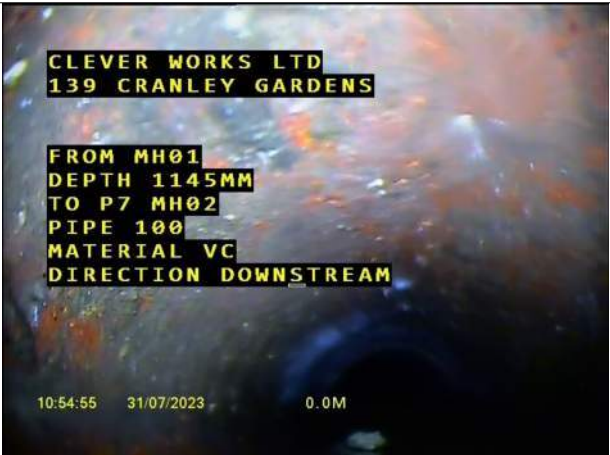
00:00:00, 0.00 m Start manhole, MH01
