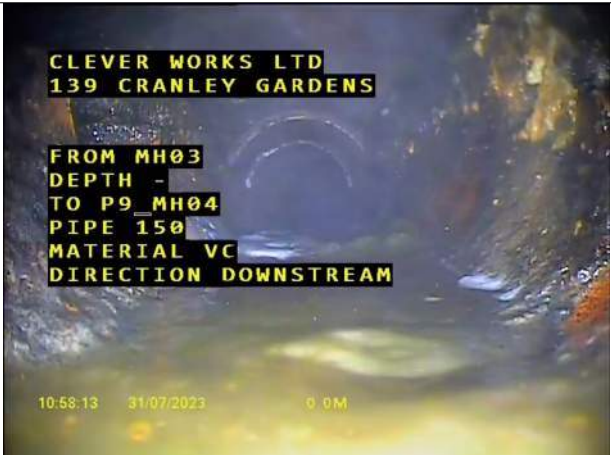
00:00:00, 0.00 m Start manhole, MH03
