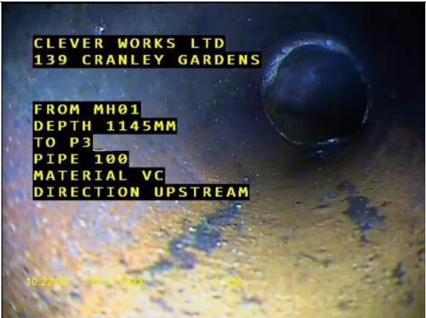
00:00:00, 0.00 m Start manhole, MH01
