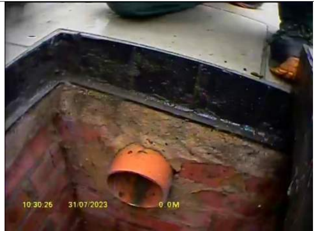
00:00:07, 0.01 m General remark, General photo for pipe identification
