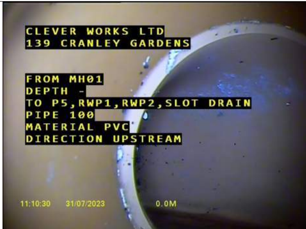
00:00:00, 0.00 m Start manhole, MH01
