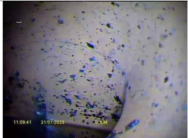
00:00:23, 0.50 m Finish gully, P6/GY3, the pipe is flowing fine, No faults
