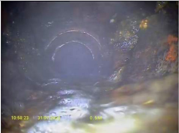
00:00:12, 0.50 m Junction at 3 o'clock, diameter: 100mm, Junction in Manhole
