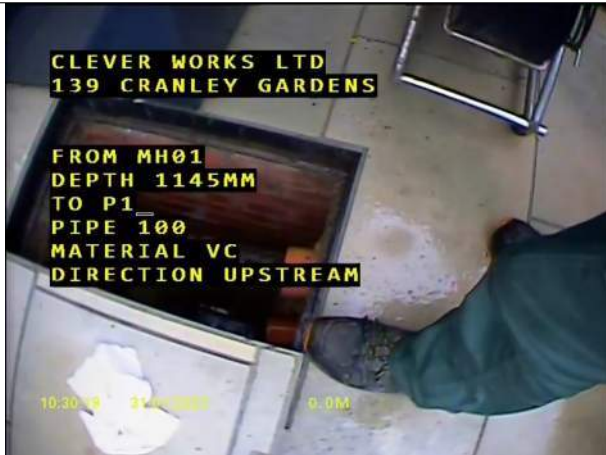
00:00:00, 0.00 m Start manhole, MH01
