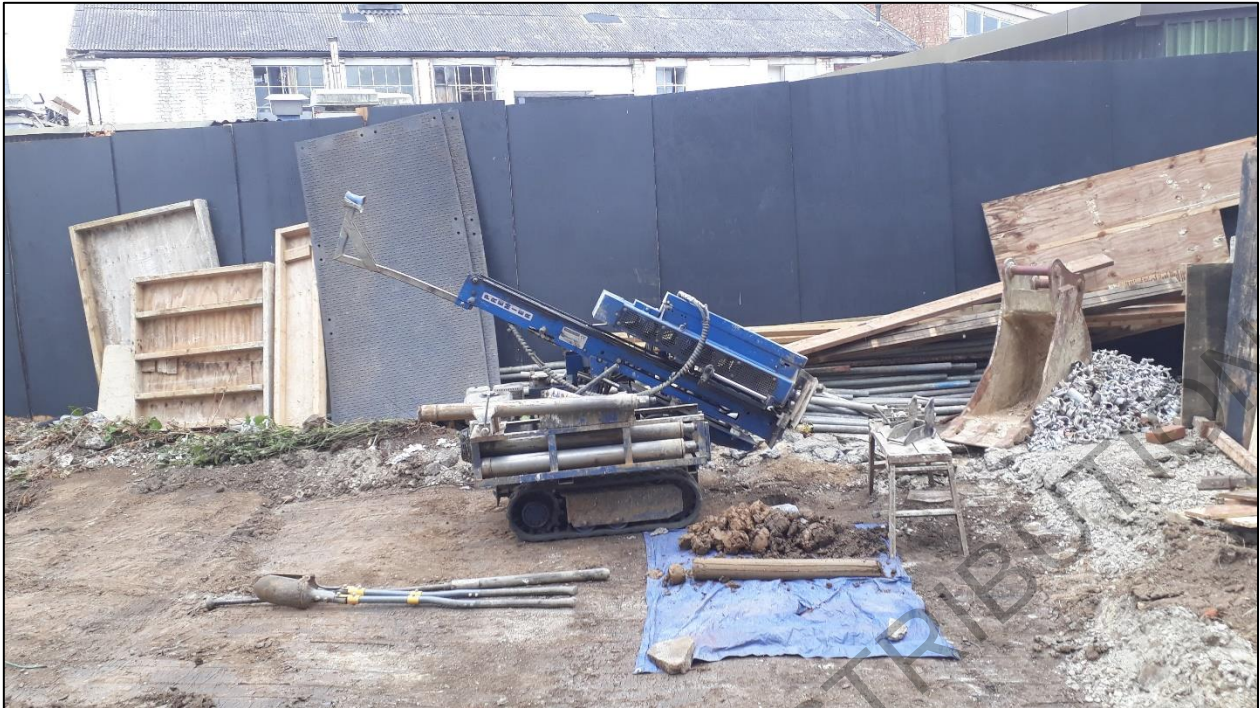
Overview of the site and the Dynamic Windowless Sampler Rig, as well as the soil encountered in BH01
