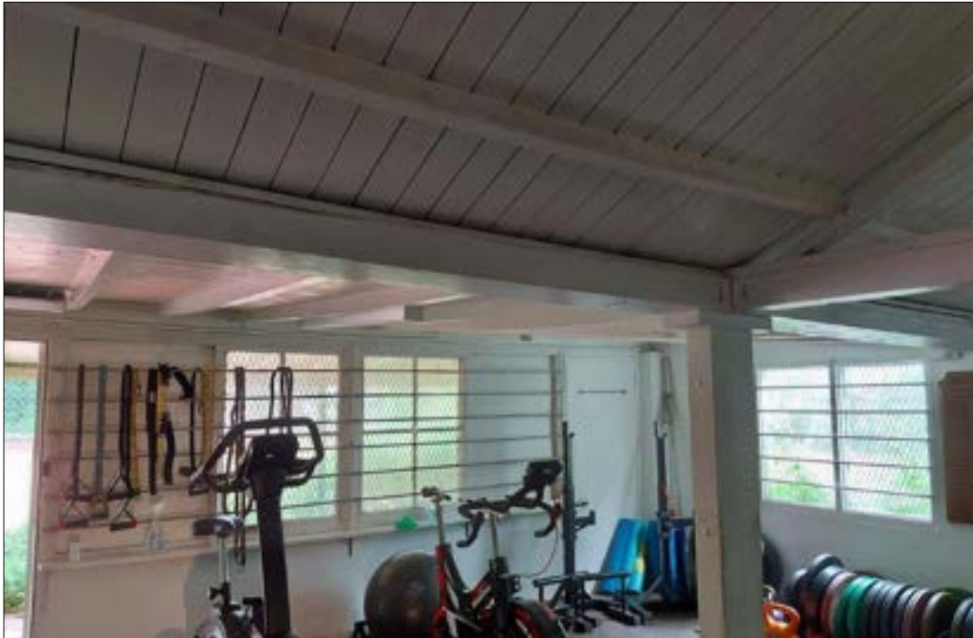
PHOTOGRAPH 3: Interior of building B2 (clubhouse)
