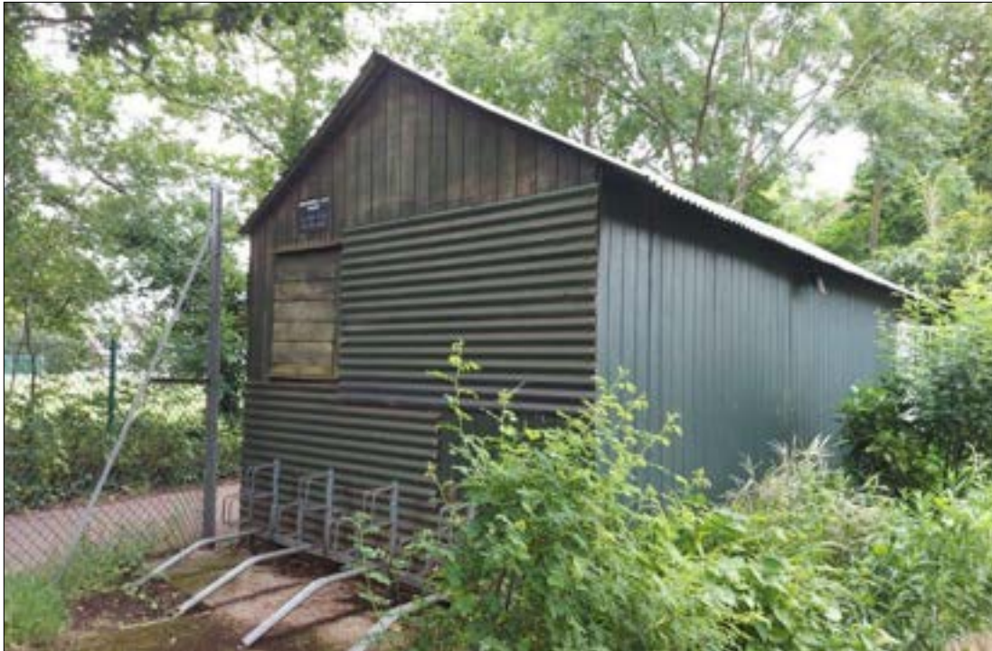
PHOTOGRAPH 1: Exterior of building B1 (storage shed)
