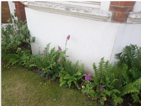
Fig 1.1: Trial Hole 1 Location
