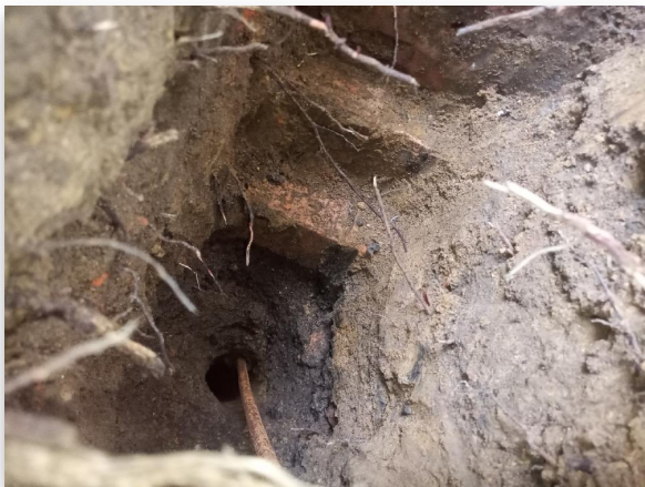
Fig 1.2: Trial Hole 1 Footing
