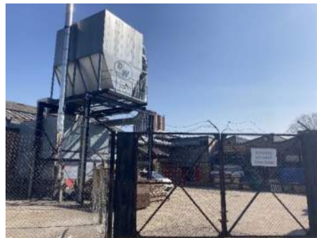
Figure 2-9 - View of DW General Wood Machinists compound, located from about 20m north.
