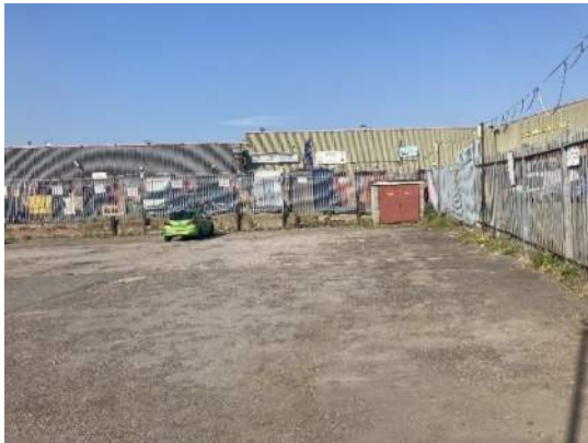
Figure 2-1 - Facing west along northern boundary of The Printworks. Electricity substation contained within brick structure.
