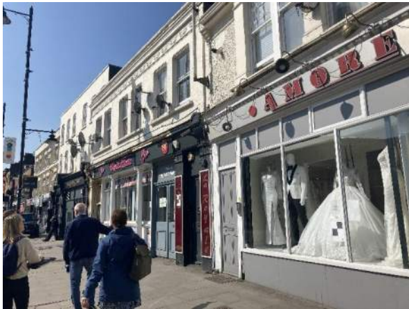
Figure 2-5 - View along the High Road, facing south.
