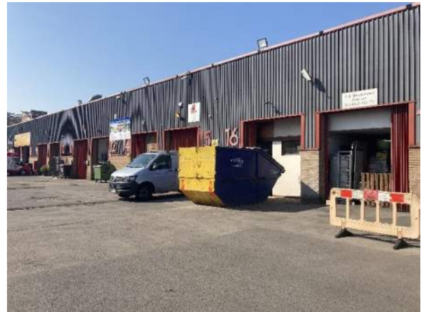
Figure 2-11 - Overview of Peacock Industrial Estate, facing southwest.
