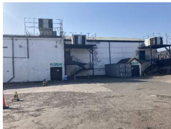
Figure 2-4 - View of western side of La Royale building, facing south.
