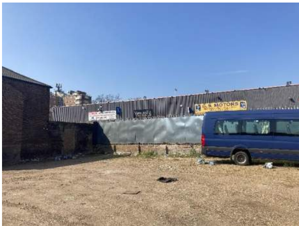
Figure 2-6 - View across southern yard area, facing west towards western Site boundary. Fly-tipped wastes evident in left of photograph.
