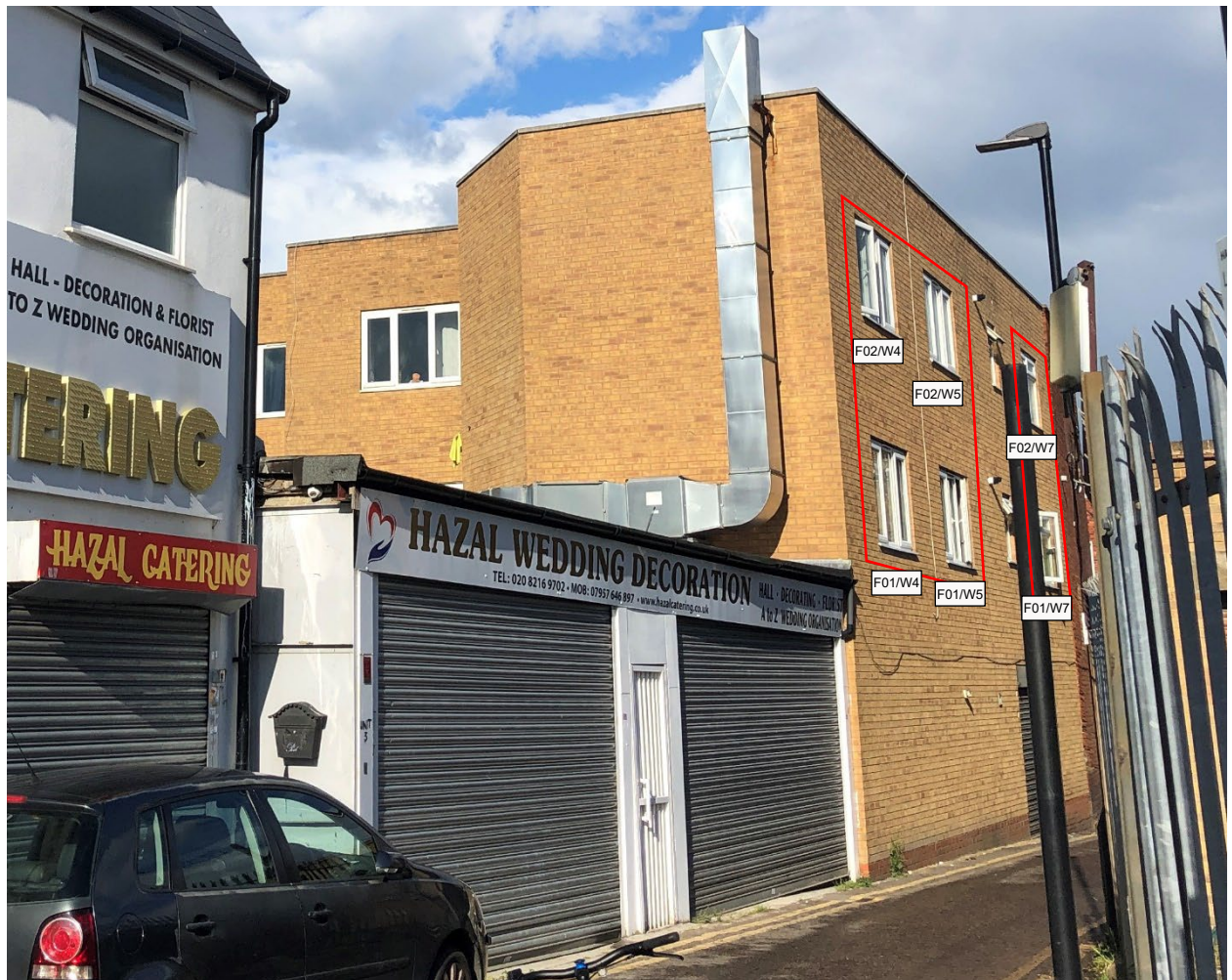
Figure 4 – Windows to living/dining rooms and bedrooms in the flank wall of 831-833 High Road are directly on the boundary with Brunswick Square facing the Site.
