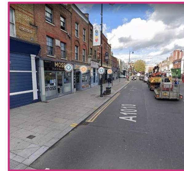
Google Streetview: High Road, looking northbound
