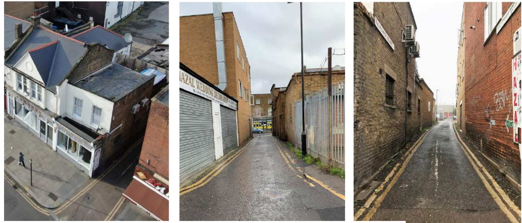
Figure 7: Photos of Brunswick Square (left to right: aerial view, view from the west, view from the east)
