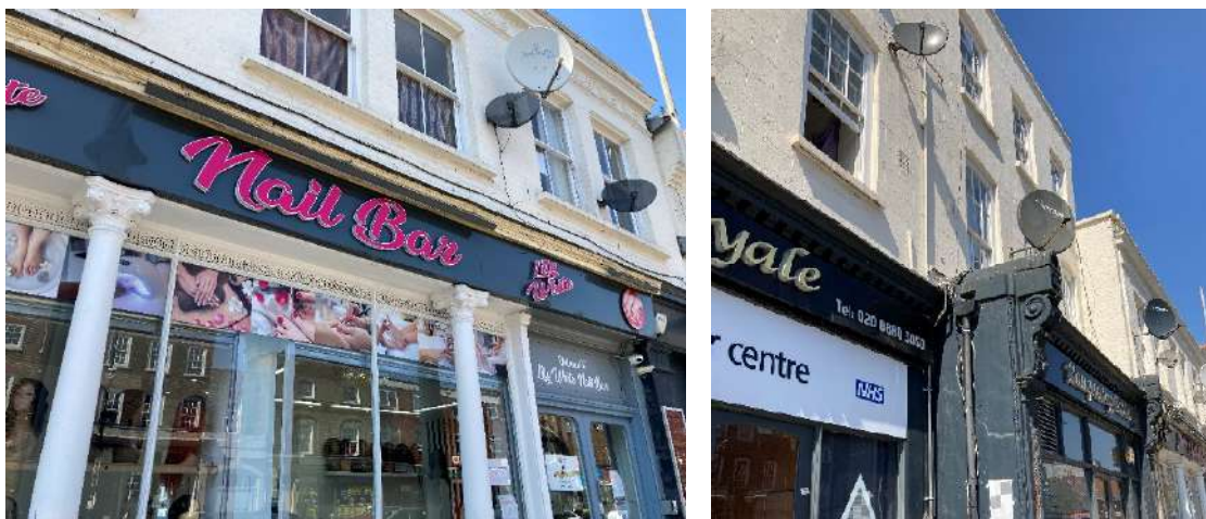
Figure 3-2 - a) pillar forming shop front to Unit 823, b) inset of Unit 821's first floor façade relative to ground floor shop front
