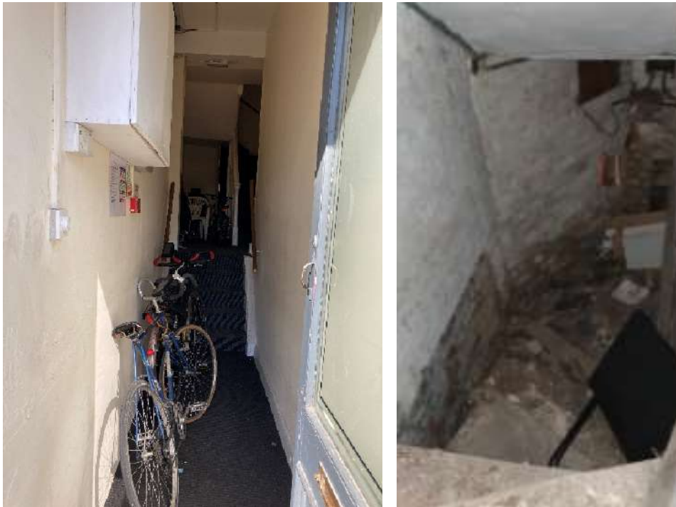
Figure 3-3 – a) Unit 819 communal hall leading to basement access, b) view of basement from ground floor access
