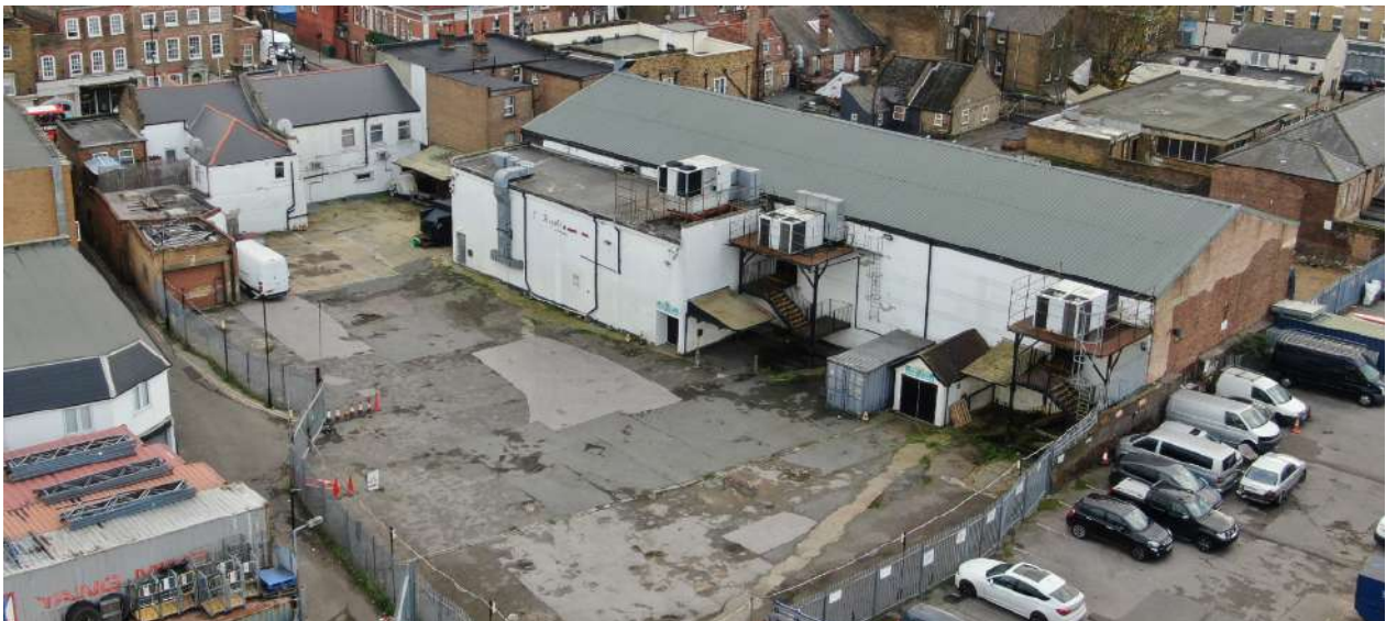
Figure 3-4 - Drone view from North-West, showing warehouse with smaller extension and steel frames in the foreground
