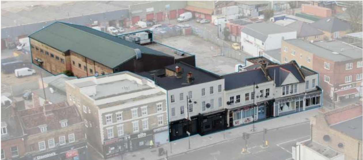
Figure 3-1 - Drone footage of existing terrace units 819-829 and extensions/warehouse behind
