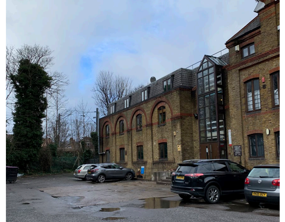
FIGURE 185. Large Commercial Building Accessed Through 551 Alleyway
