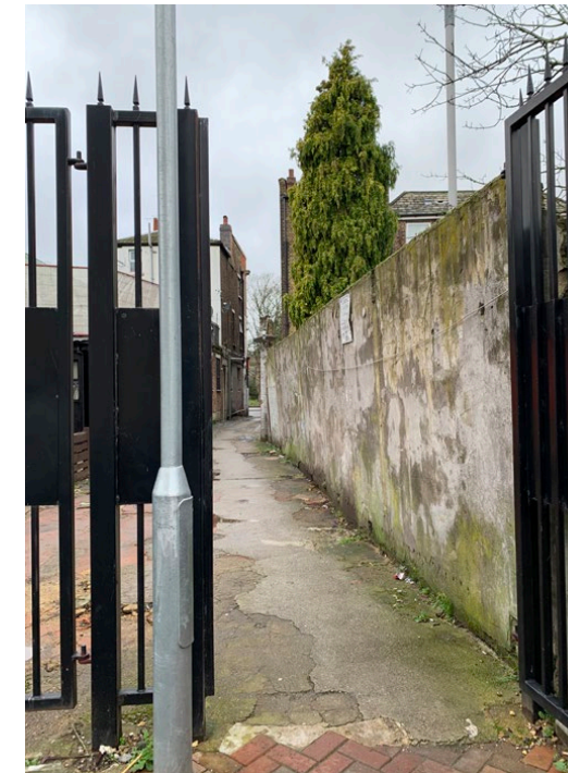
FIGURE 195. Access to the HR from Resi through the Alley
