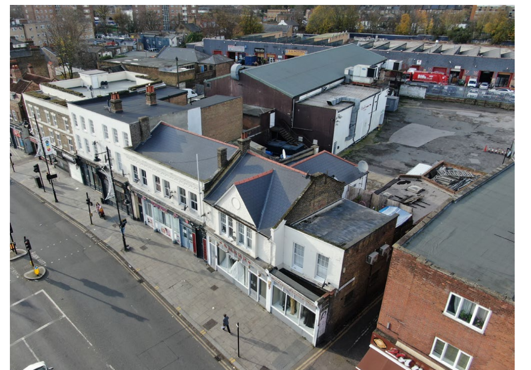
FIGURE 9. View looking south west from the High Road (4)
