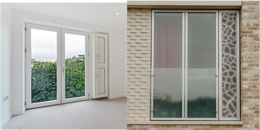
Figure 6—9 Operable attenuated louvre
