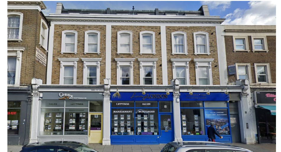
FIGURE 148. Example of compliant shop fronts in Tottenham
