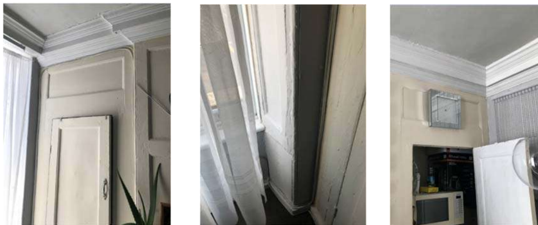
Figure 33 – (left) moulded cornice, bead panelled panelling and cupboard door, (centre) panellled window reveal (in abraded and poor condition), and cornice, cupboard and panelling symmetrical to the cupboard on the left.
