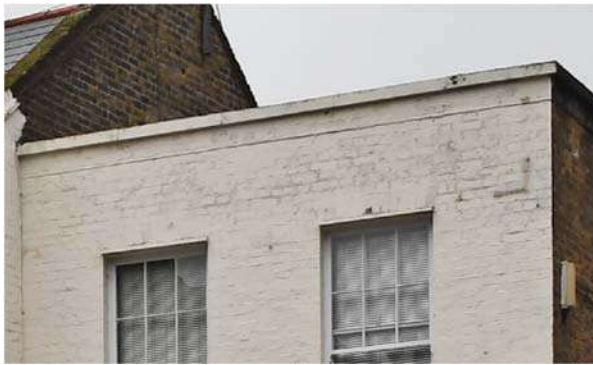
Figure 65 (left) – damp at high level of the frontage beneath the modern paint.
