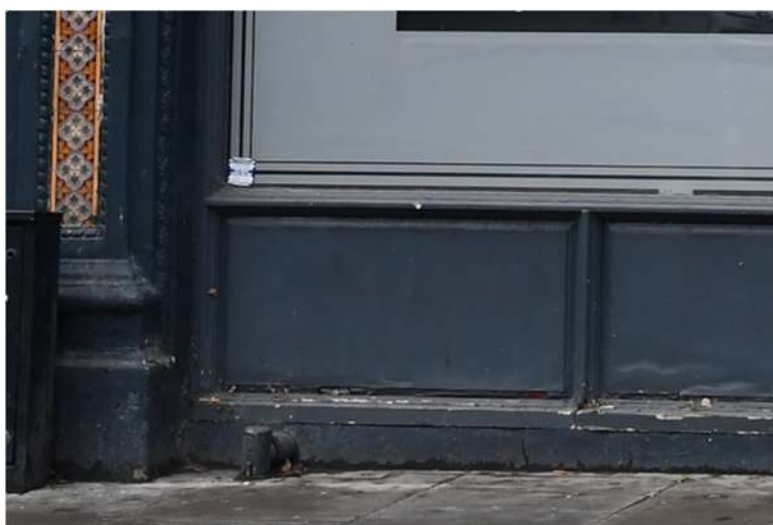
Figure 52 (above left) – Thick layers of cracked paint over the original green glazed tiles.
