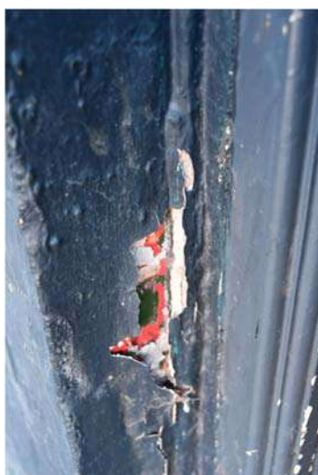
Figure 52 (above left) – Thick layers of cracked paint over the original green glazed tiles.
