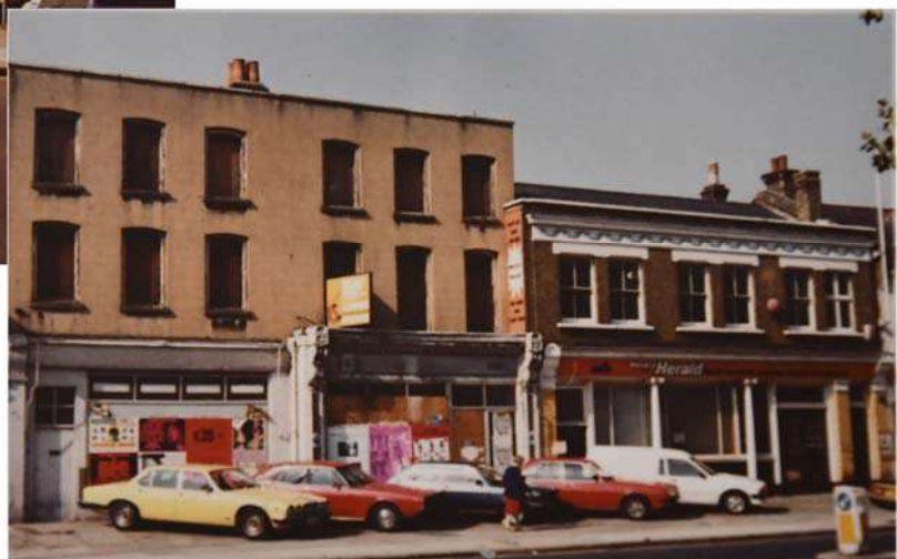
Figure 19 (below): 819-821 High Road boarded up in c. 1980 - Haringey Archive Bruce Castle.
