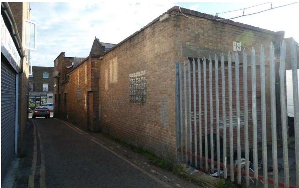
Figure 85 - The rear of 829 High Road, from Brunswick Square.
