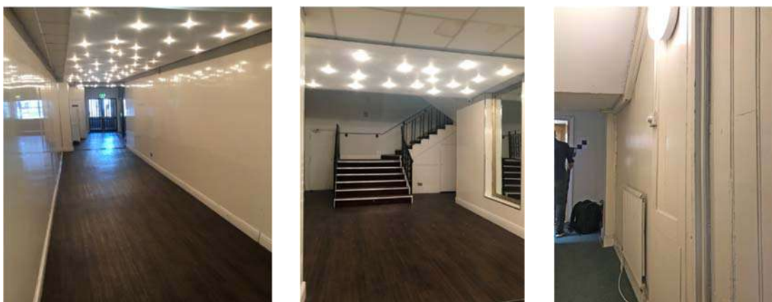
Figure 32 – (left and centre) Interior of circa 1993 with suspended ceiling and claddings. (right) C19 stair, bead boarded stair enclosure and likely C18 reused door.
