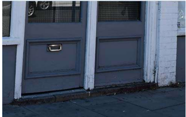
Figures 60 (left) and 61 (right) – water damage to joinery at plinth level
