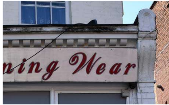
Figure 65 (left) – damp at high level of the frontage beneath the modern paint.
