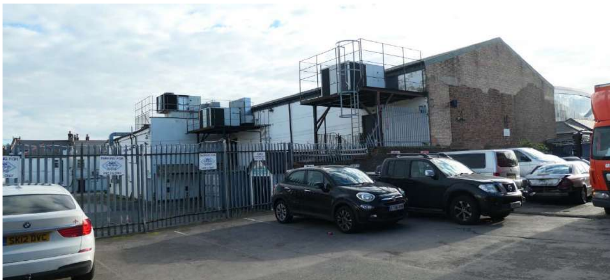
Figure 75 - The shed at the back of 819-821 High Road, and the northern part of the Site, from the NW.
