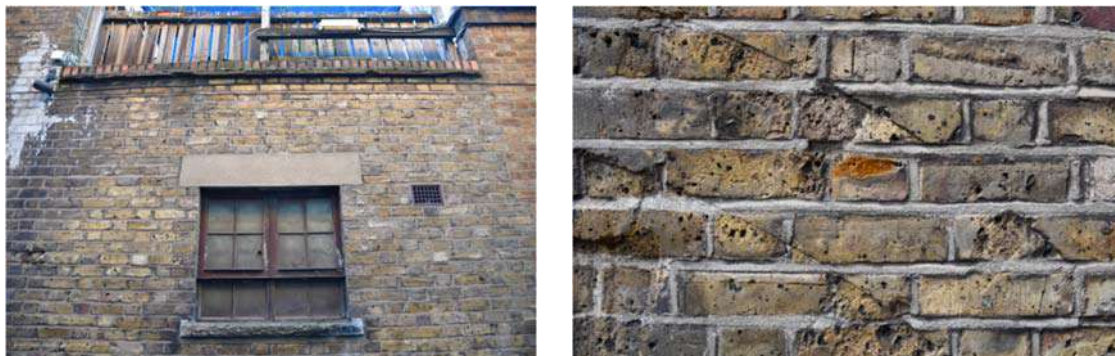
Figure 49 (left) – Typical reused iron window with concrete head and cill. This rear extension is built in the early C20 at the same time as the front element. On the far right, the bricks of the 1980s garage extension are visible.
