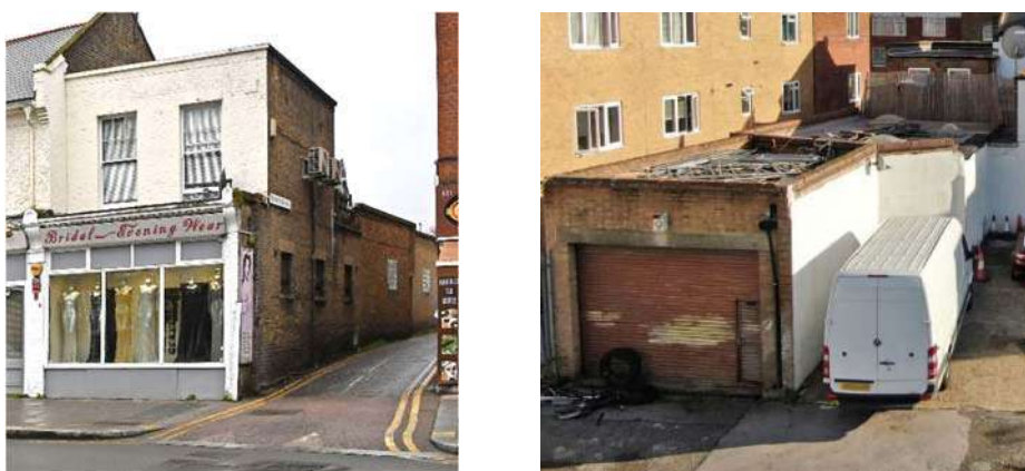
Figure 45 – Front. Figure 46 – Rear elevation of 829 High Road.
