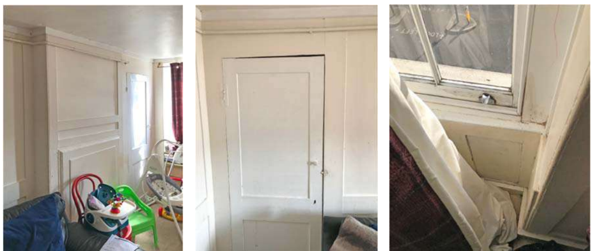
Figure 31 – (left) C18 plain panelling, fire surround and cupboard door (centre) detail of 2-panel cupboard doors with H hinges, simple doorknob and turnbuckles, and (right) window sash and panelling.
