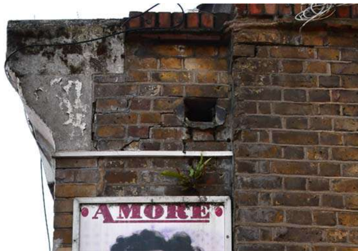
Figure 66 (right) – damp staining of shopfront. Damage to outer edge of console.
