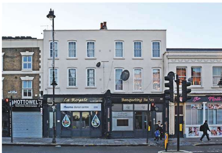
Figure 25 – Frontage of 819-821 High Road.
