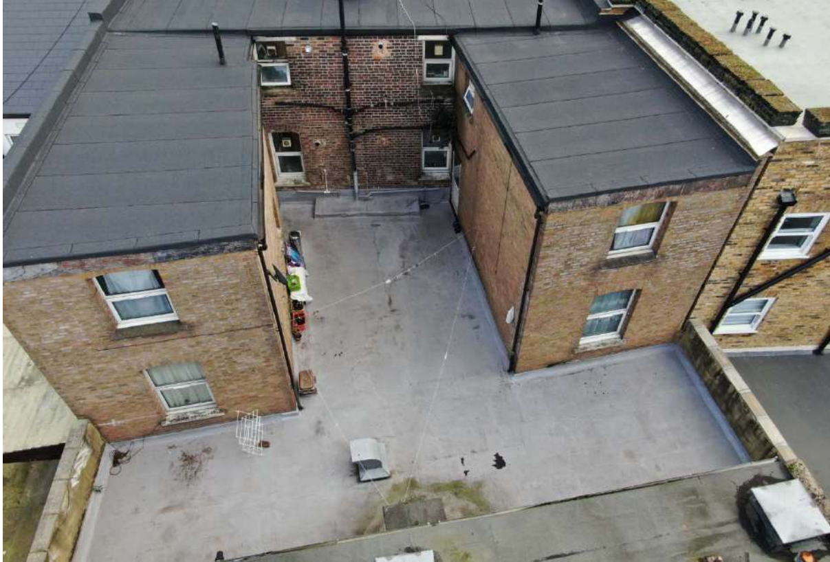
Figure 72 – An aerial view of the back of 819-821 High Road, showing the single storey extension/link with the shed to the rear.
