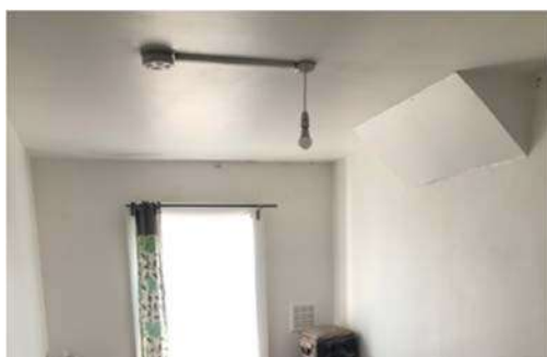
Figure 37 – (above) south-east room with fireplace removed.
