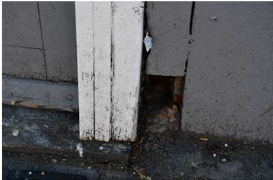
Figures 60 (left) and 61 (right) – water damage to joinery at plinth level
