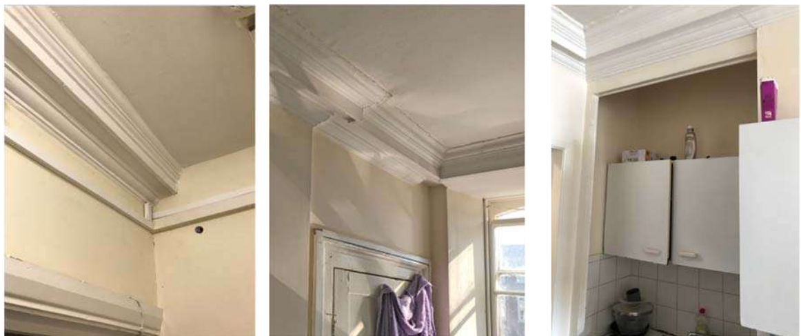
Figure 30 – C18 moulded cornice with (left) typical C20 doorway in hall, (centre) C18 cupboard door and architrave, and (right) former cupboard.
