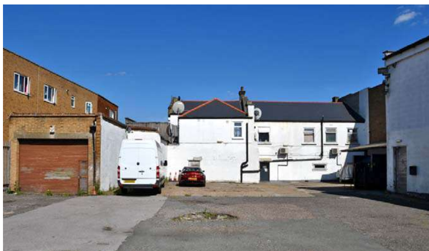
Figure 51 – From the boundary of the conservation area, looking towards the Rear elevations of 823-829 High Road. Far right are the large C20 rear extensions to the listed buildings 819-821 High Road.
