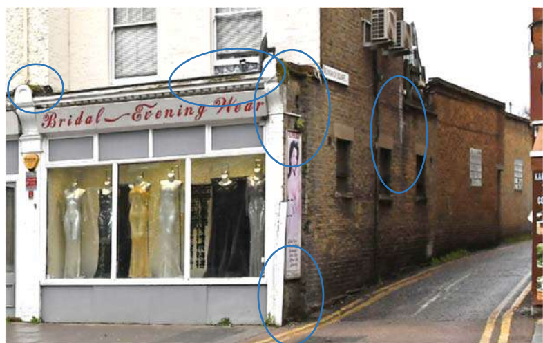
Figure 64 (right) – staining and plant growth on the north-east corner (circled)
