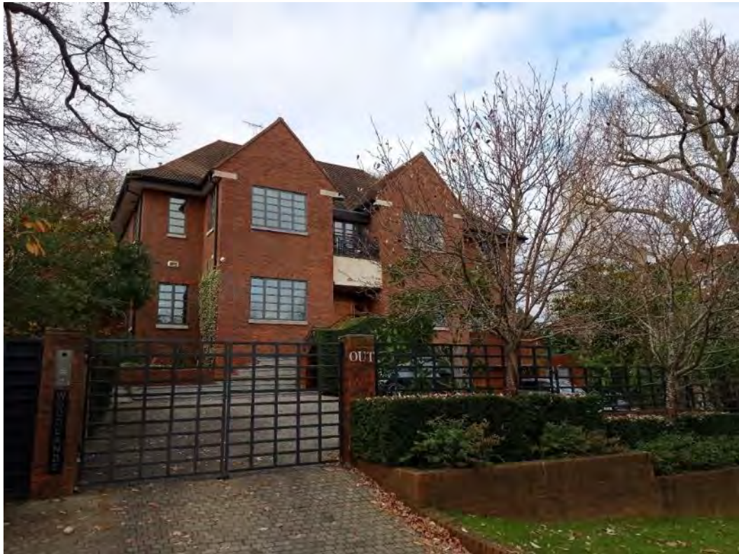
Figure 22: Woodlands; original house demolished and replaced in 1997 in rather bland format
