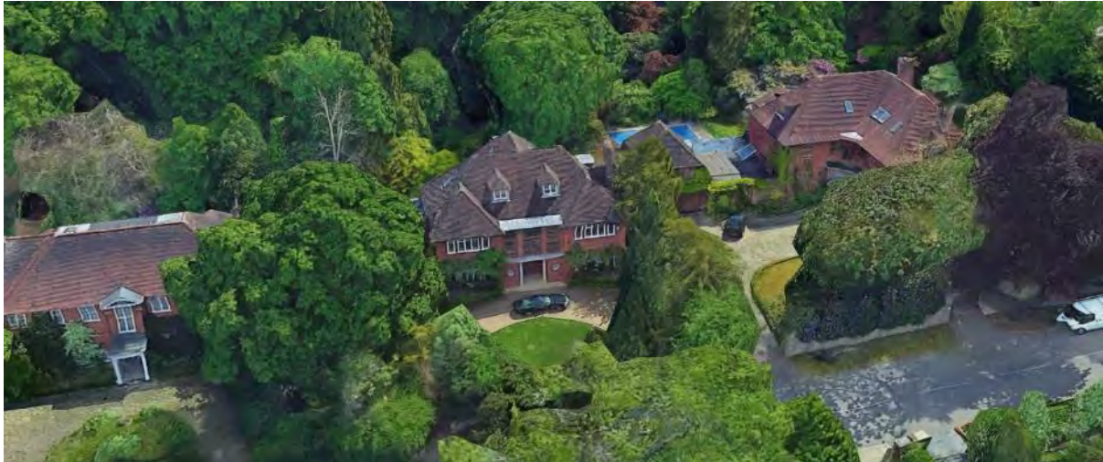
Figure 39: Aerial view of Bracken Knoll from the west
