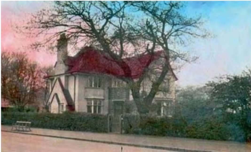
Figure 17: No. 32, Hampstead Lane in 1927 – called ‘Wood Edge’ as it marked the eastern periphery of what was the Bishop’s Wood, mostly wiped out by the developments of Courtenay Avenue, The Bishop’s Avenue and Sheldon Avenues in the 1920s and 1930s
