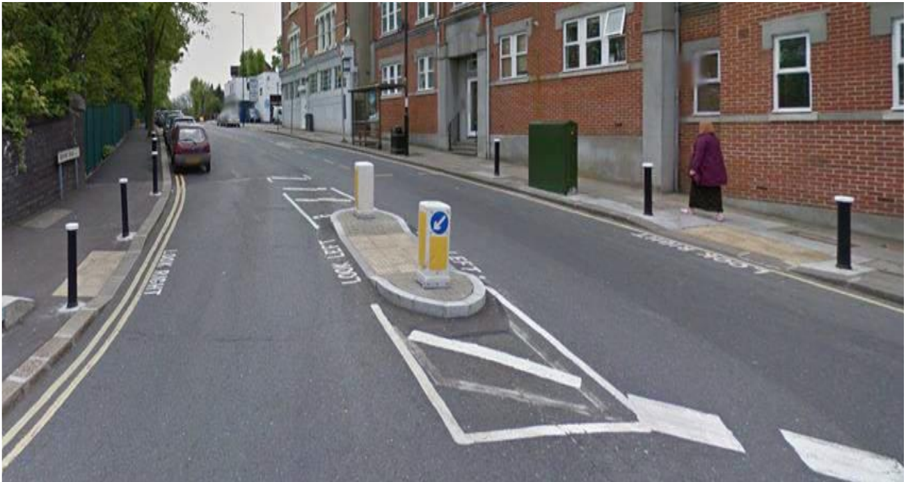
Fig 3 Pedestrian Island at the junction of Bedford Road/Buckingham Road/ Crescent Road
