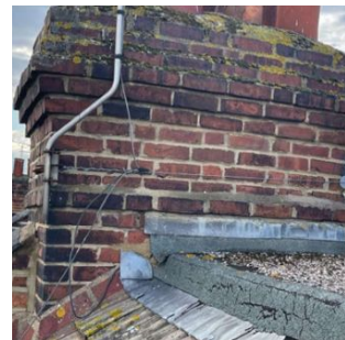
Failing condition of external wall to LGF/Existing flat roof to dormer/Existing flat roof/tile roof that needs replacing 41 Grand Ave - Design & Access Statement
