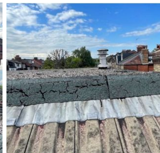
Failing condition of external wall to LGF/Existing flat roof to dormer/Existing flat roof/tile roof that needs replacing 41 Grand Ave - Design & Access Statement
