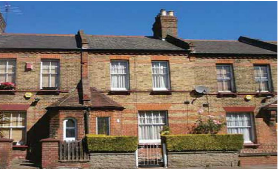
Photo 2: Moselle Avenue Front Elevation
