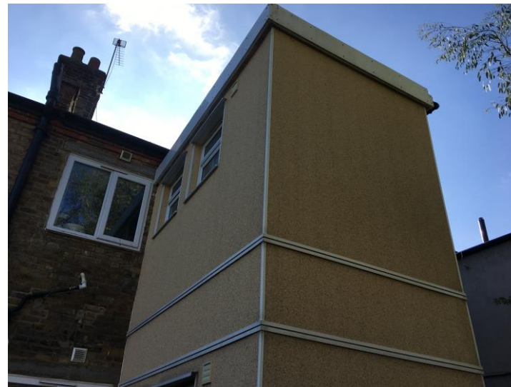
Photo 4: 183 & 183a Gladstone Avenue double storey pod.
