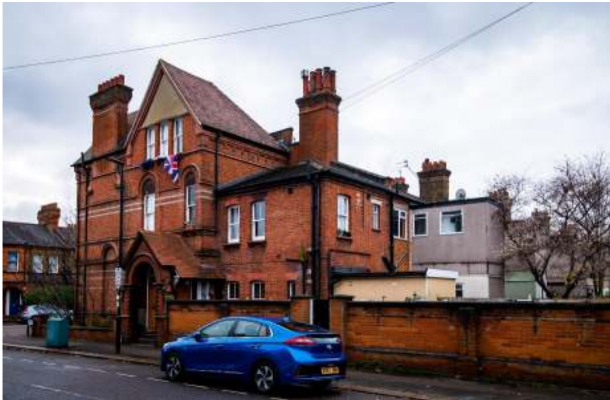
Figure 43: View of rear extensions along the north side of Gladstone Avenue. Their design and detailing is characteristically modern and in contrast with the architectural character of the host building. However, due to their uniformity and almost ubiquitous nature within the CA, they add another layer to the historic and architectural significance of the conservation area as a whole. However due to their age, weathering and relatively non-permanent construction, they appear to have served their lifespan and are in need of replacement.
