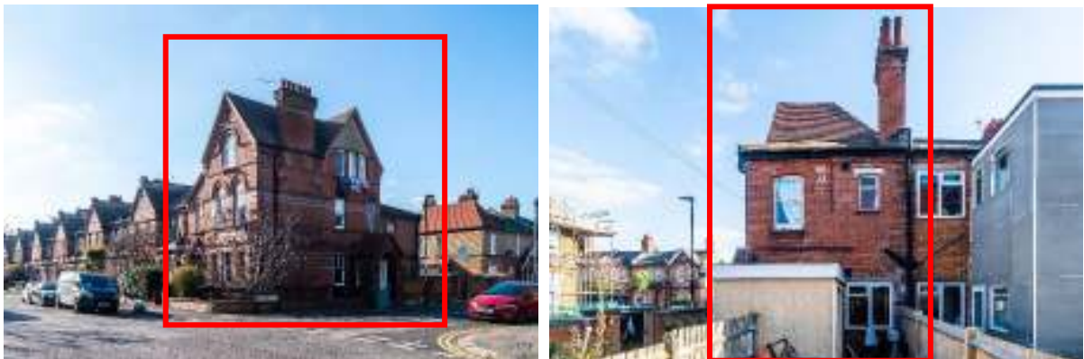
Figure 51 The photos showing the south elevation(left) and the north elevation(right) of nos. 221 & 221A (highlighted in red).
