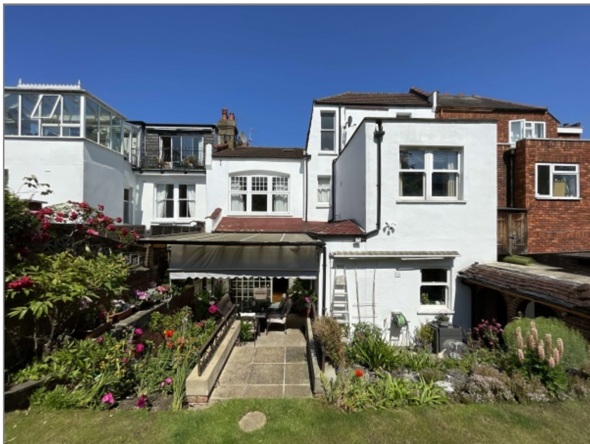
View - Neighbours Rear Elevation
