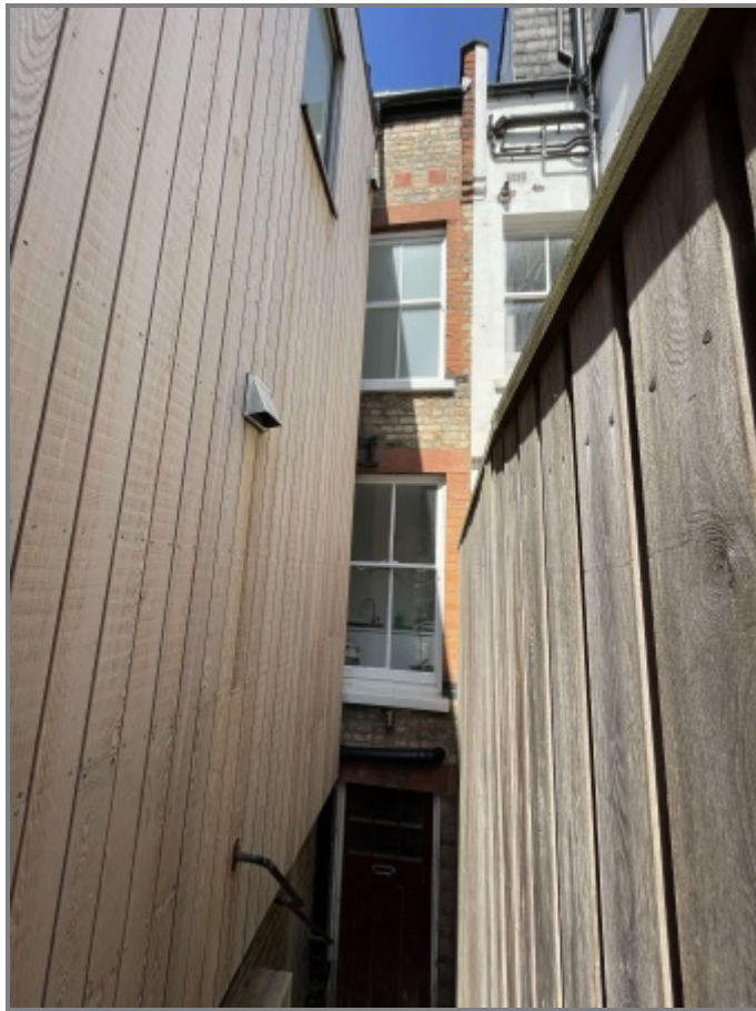
View - Neighbours Rear Elevation
