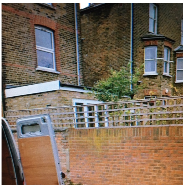
Full width extension to 17 Church Lane
