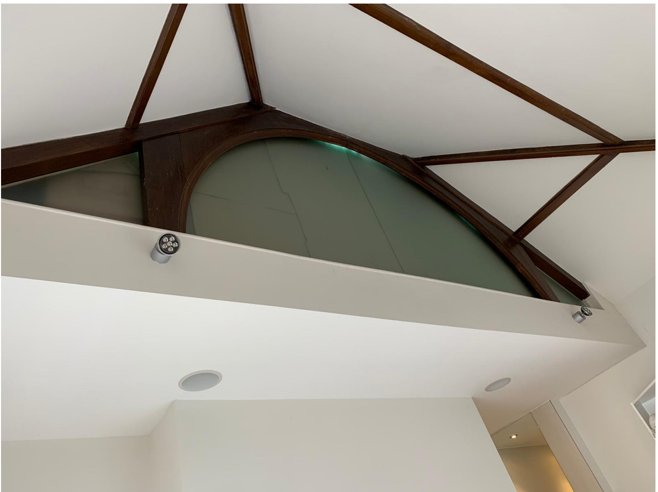
Image 1 : Modern cladding over heritage structure to be removed
