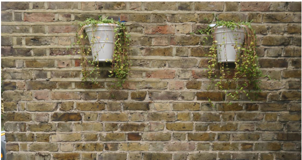
(A) Existing Brick
