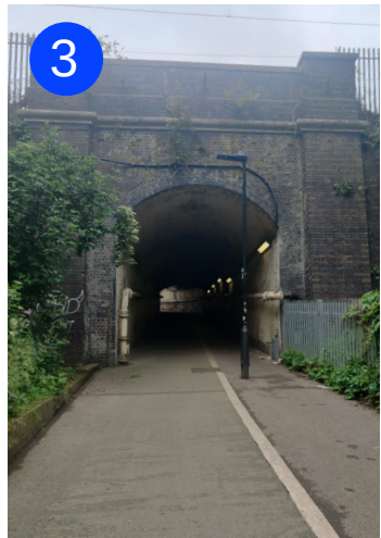
Penstock Foot Tunnel
