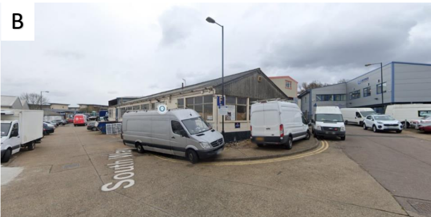
The view along Ring Way, facing south-east, showing Block F.
