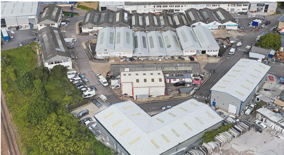
View Facing North
