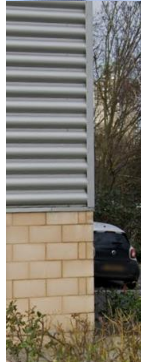
Brickwork Plinth
