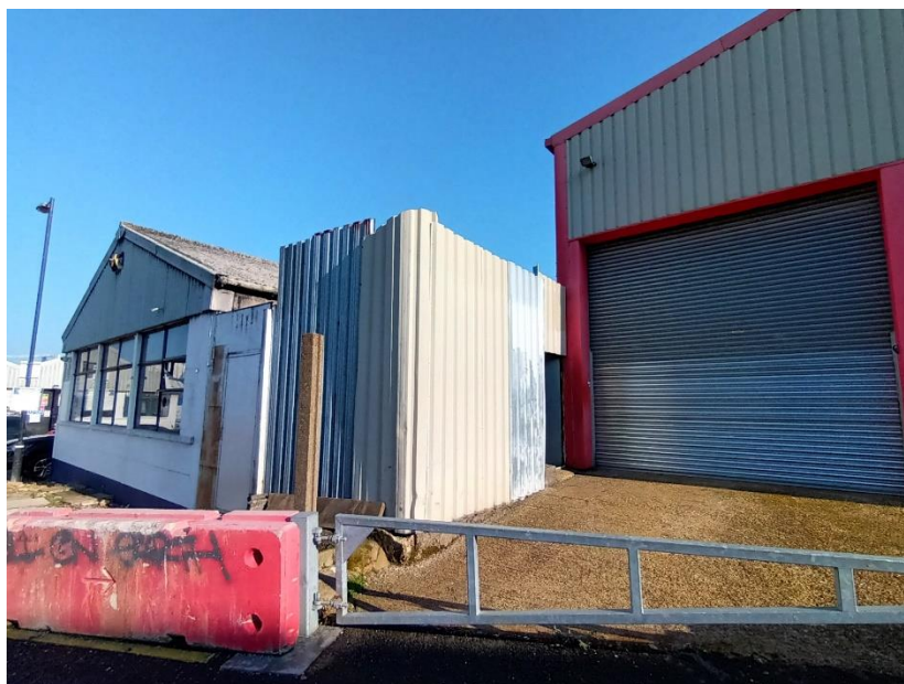
Photo 2. South-west corner of buildings, looking north-east
