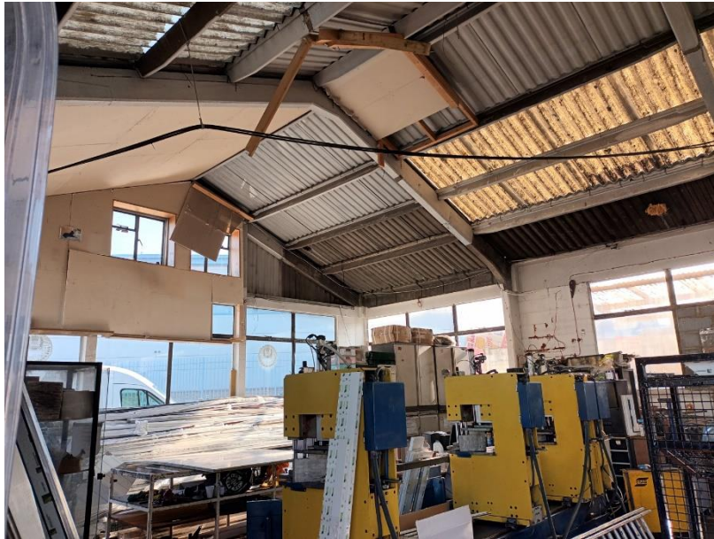
Photo 3. Interior of one of the industrial units. Note lack of potential roost features for bats and the well-lit and disturbed conditions, creating negligible bat roosting potential within.
