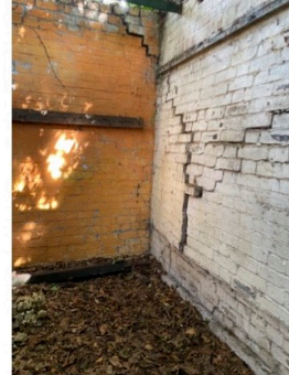
Boundary wall to southern boundary (to north of T1)
