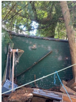
Sunken form (up to 500mm) of previous garden building / greenhouse
