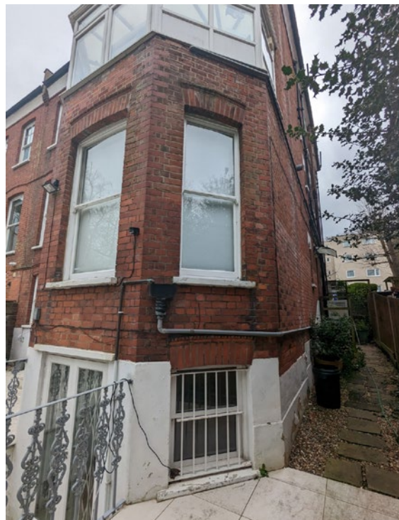
The existing rear bay window and pumped external drainage along the rear / side of the property. The proposal is to remove the drainage, handrail and infill the patio stairs down.
