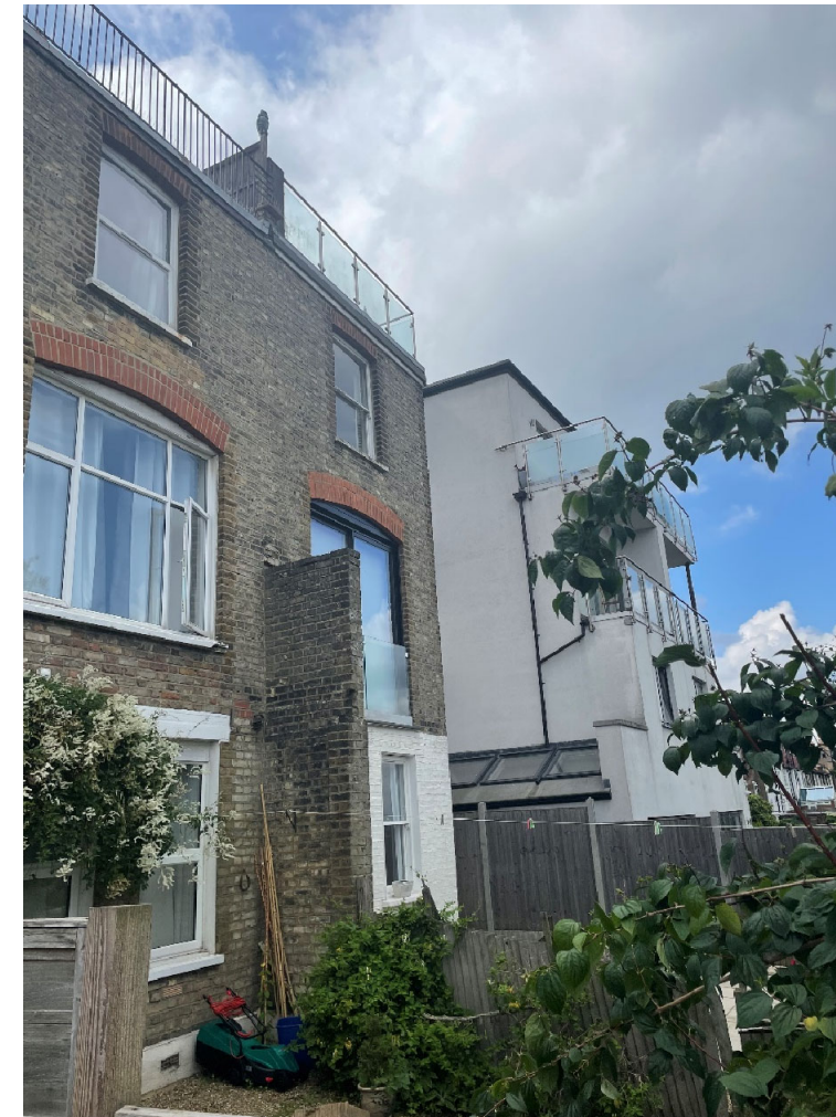
Rear elevation of 229 & the block of flats / 227 APR.
