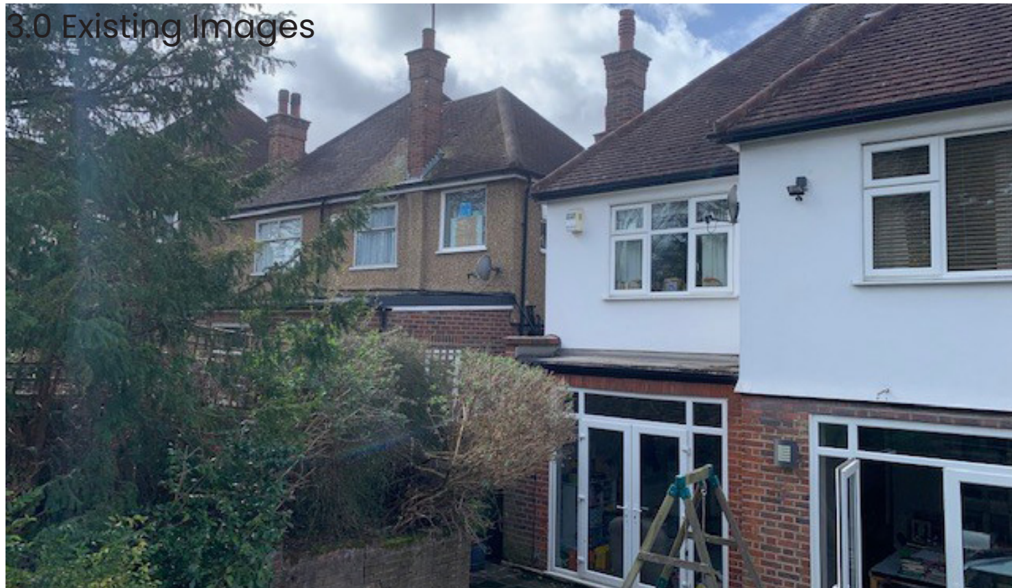
1. Existing rear elevation looking left to No.40 Ringwood Avenue
