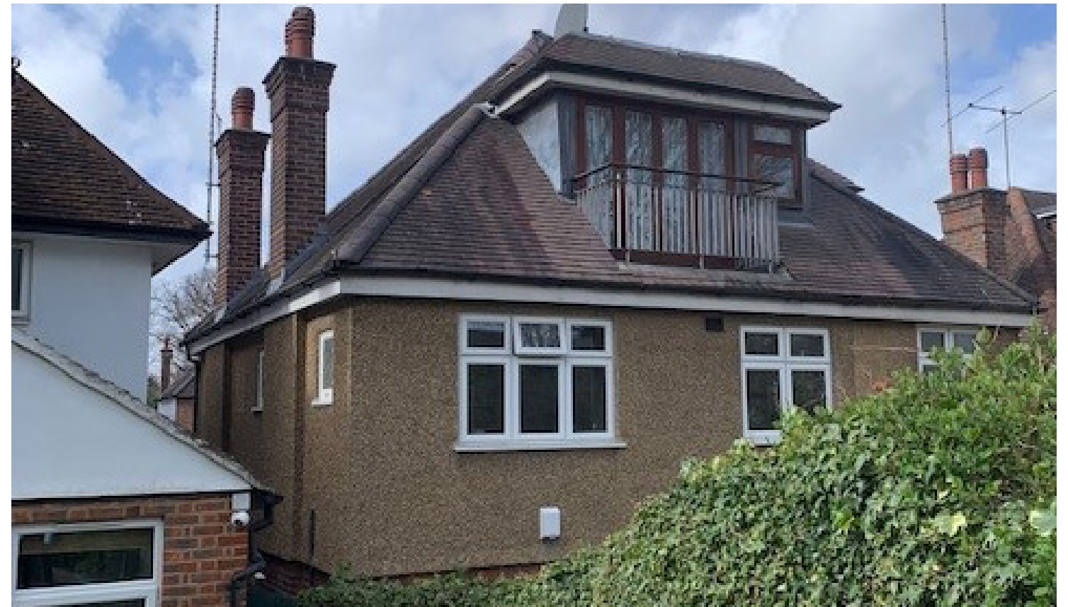
2. Existing rear elevation looking left to No.36 Ringwood Avenue
