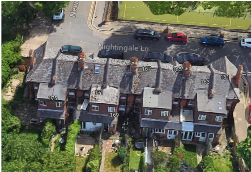
Two storey extensions built to entire terrace
