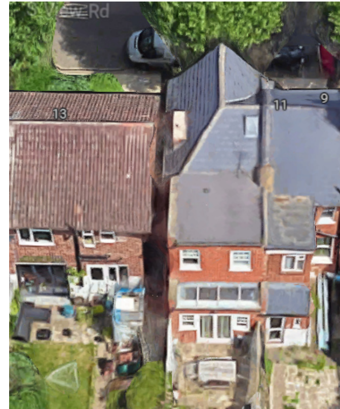
11 South View Road – Two storey rear extension with additional single storey ground floor
