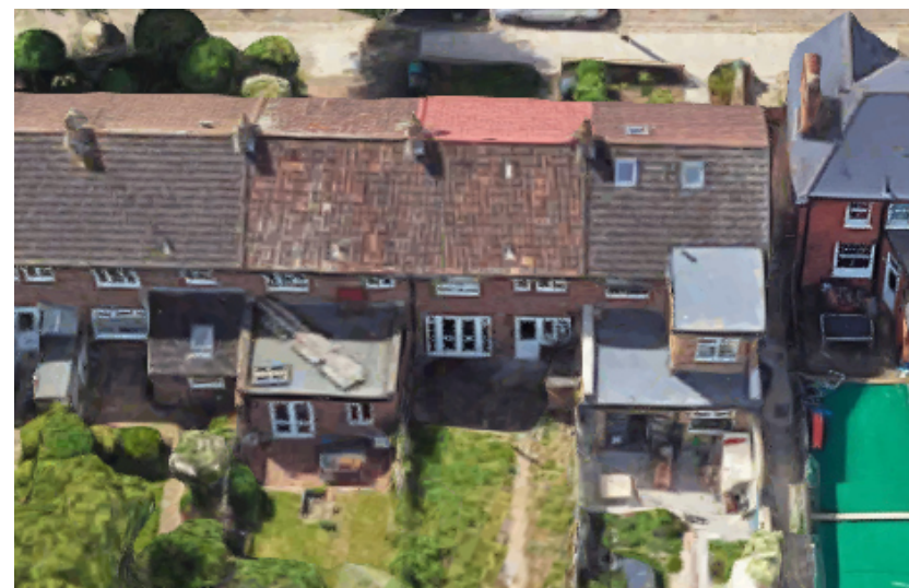
Rear elevations of South View Road – Large extensions and two storey extensions
