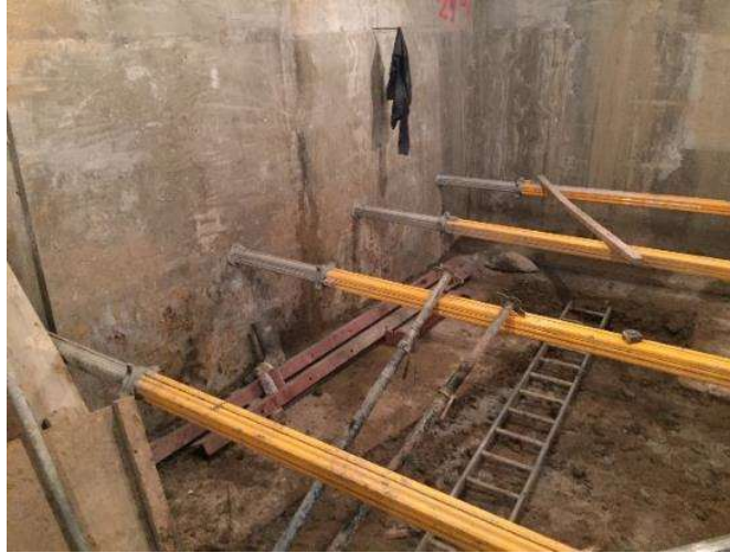
Figure 26: Example of propping (relevant to main basement)
