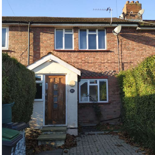
Figure 10 - No.121 Coppetts Rd - front view
