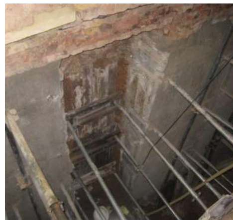
Figure 25: Examples of propping (relevant to excavations close to and below existing building)
