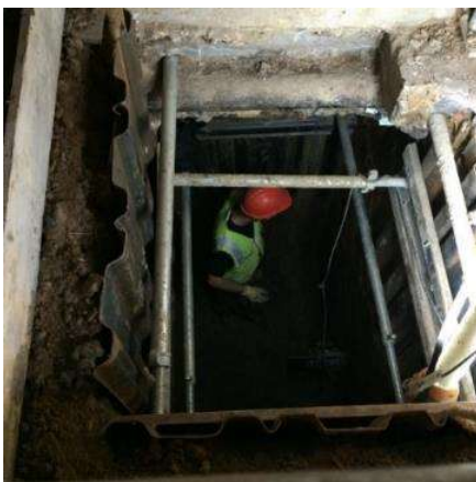
Figure 25: Examples of propping (relevant to excavations close to and below existing building)
