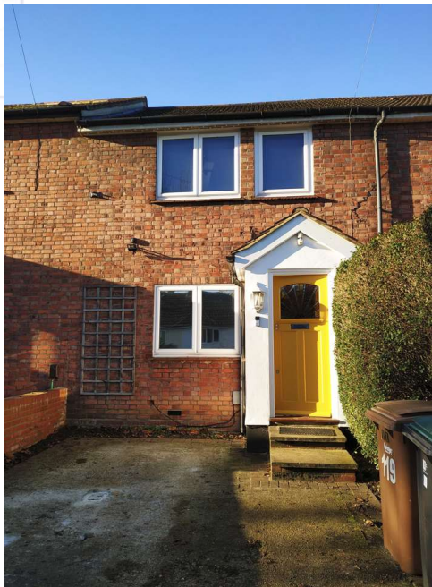
Figure 5 - view of front elevation
