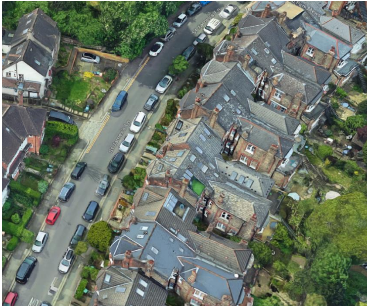
Above: Gable walls to properties within St Jame's Lane
