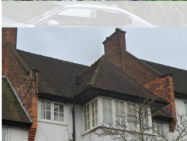
Above: Brick detailing to replicate to raised end wall
