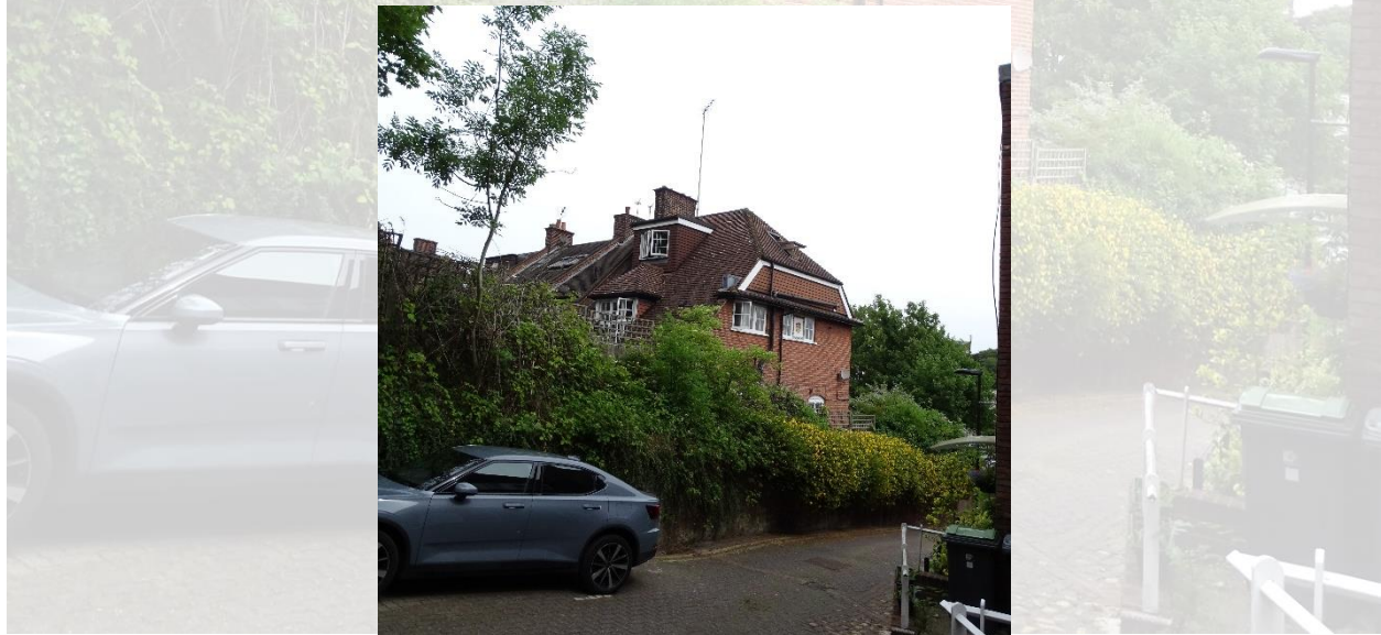
View of the rear and side fenestraion of No.34 St Jame's Lane
