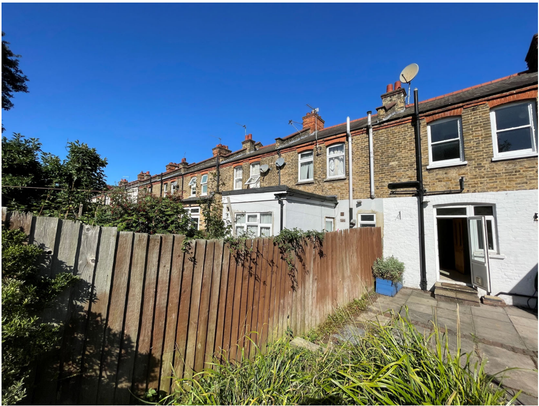
View of the rear / side boundary
