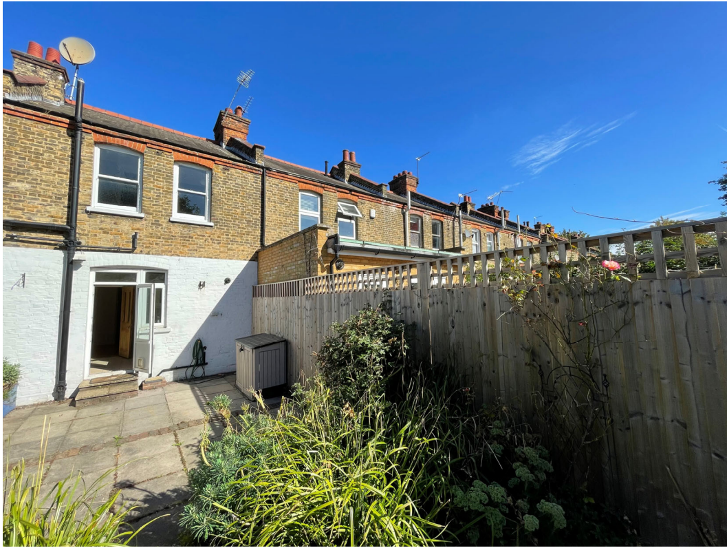
View of the rear / side elevation
