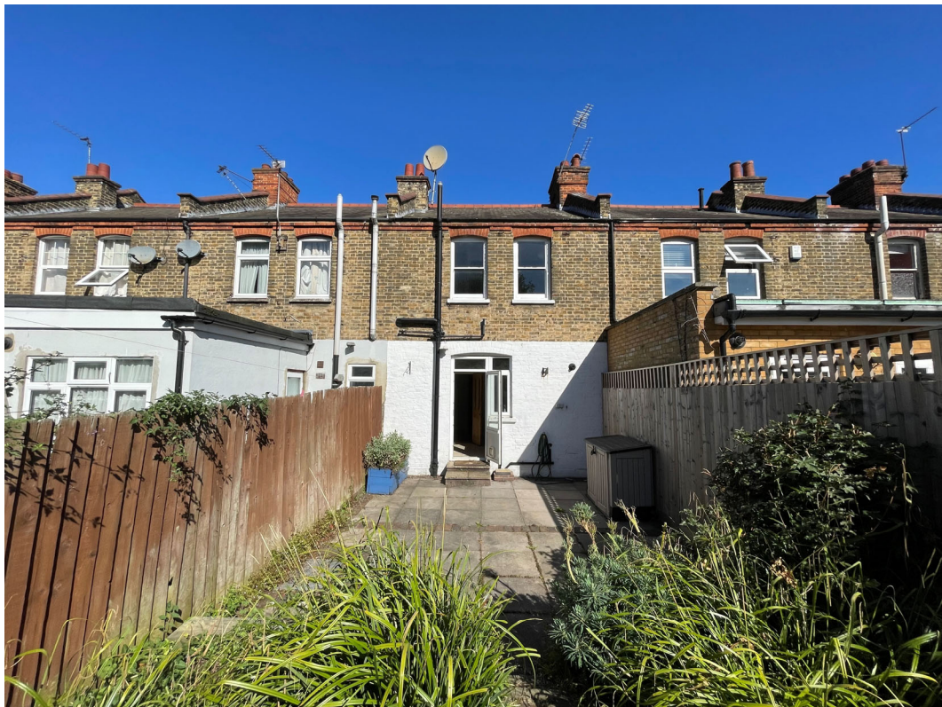
View of the rear elevation
