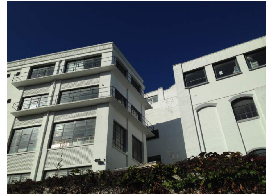
The South East elevation showing the range of external textures on the building
