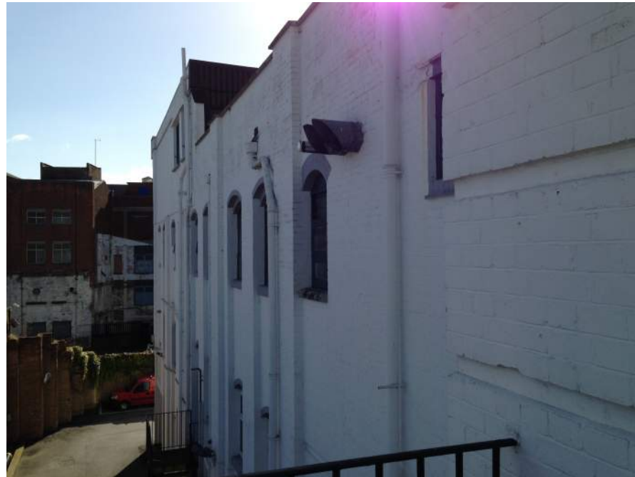
The North elevation showing the brick detailing recesses and columns. Both internal and external masonry features are a key part of the building character.
