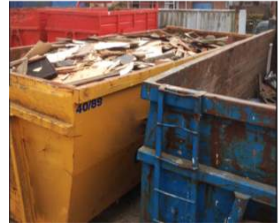
Site waste managed into separate streams
