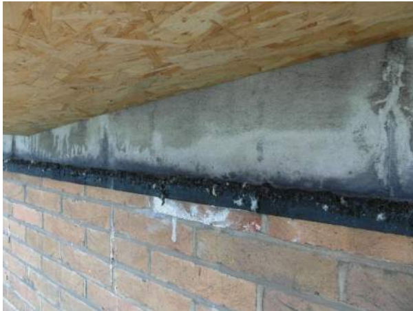
Photo 45: Cornice at third floor showing exposed vertical concrete face, and lead flashing above brickwork (1)
