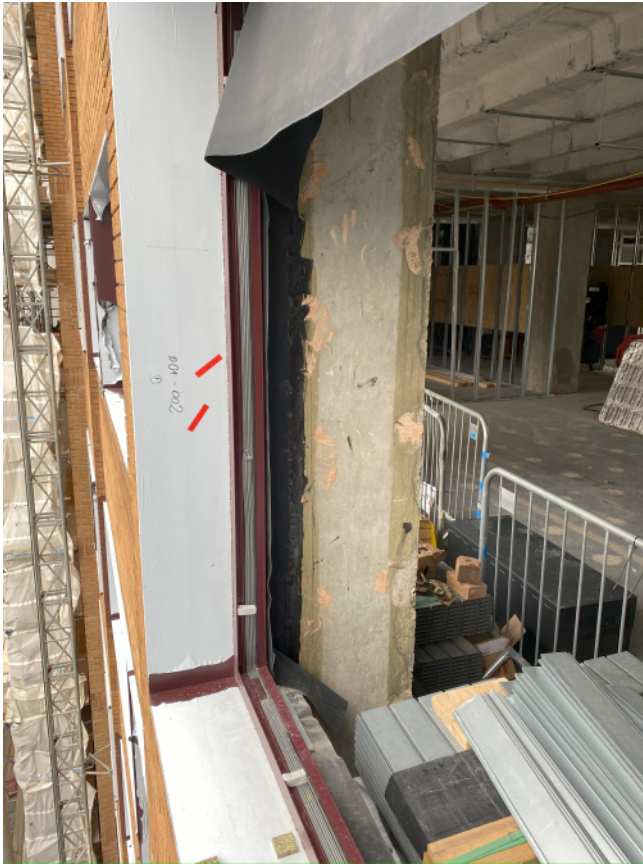
Existing photo showing, retained brickwork, window installation and internal insulation to concrete column.
