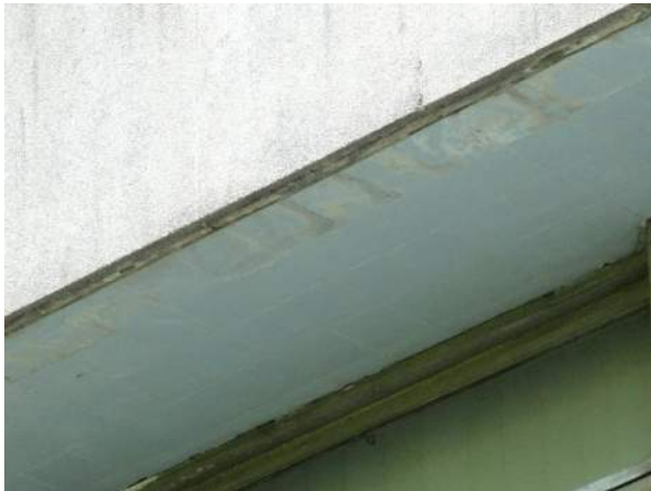
Photo 53: Tiled area at West wing building – not accessible for close inspection
