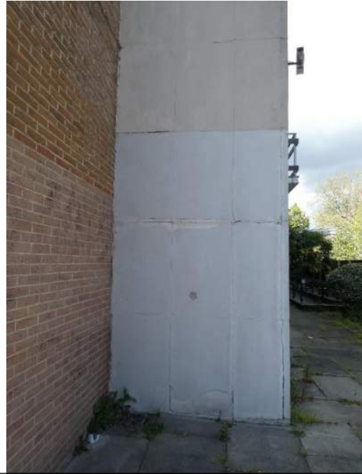
Photo 18: Lighter colour concrete panels at South-East corner, with skewed joints in render
