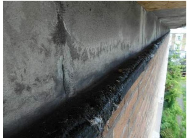
Photo 46: Cornice at third floor showing exposed vertical concrete face, and lead flashing above brickwork (2)
