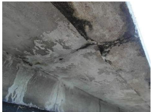
Photo 48: Water run-off on stone cladding above brickwork
