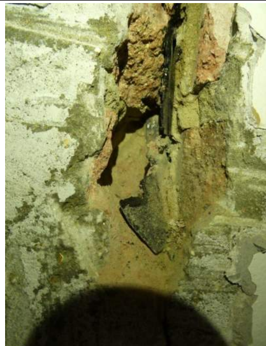
Photo 32: Intrusive investigation R1 at movement joint internally with bituminous membrane and compressible board
