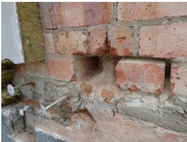
Photo 23: Intrusive investigation location P1, outer face of inner brickwork leaf, and steel fixings
