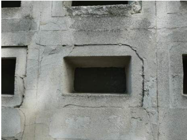
Photo 21: Punched windows in precast concrete panels on West elevation (with some glazing replaced with wooden sheets)
