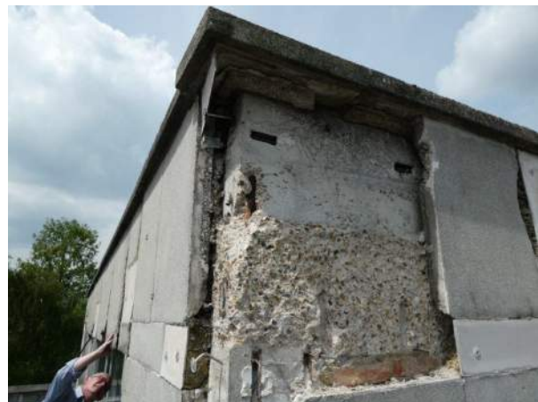
Photo 24: Intrusive investigation location P2, concrete behind with cast-in channels and concrete fill in cavity
