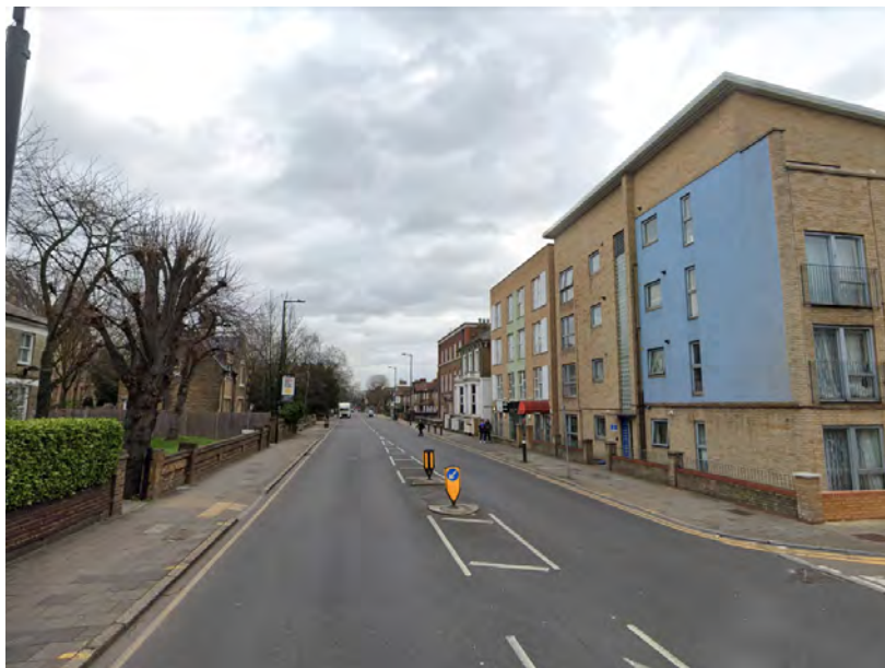
View east along Lordship Lane, with the site seen in the centre of the image
