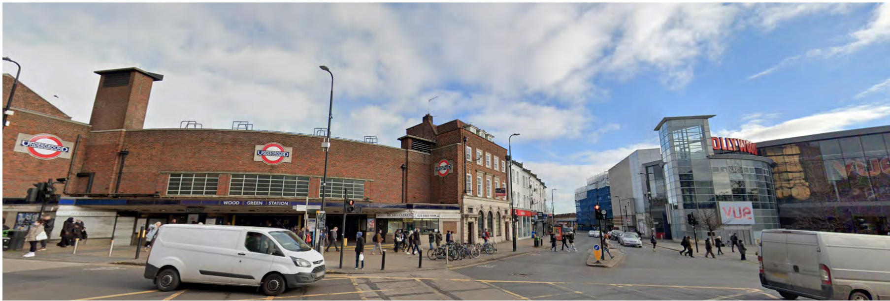
Panoramic view showing Wood Green Station and the entrance to Lordship Lane
