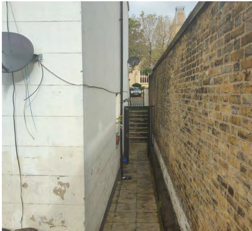
(6) Existing steeply stepped access to rear courtyard
