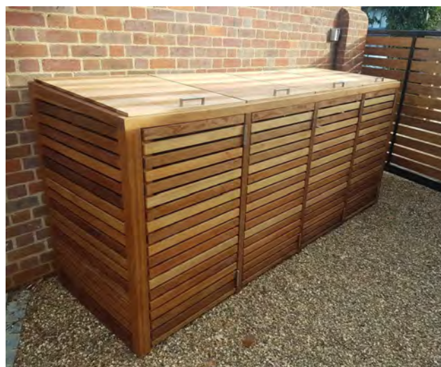
Example of timber slated bin store
