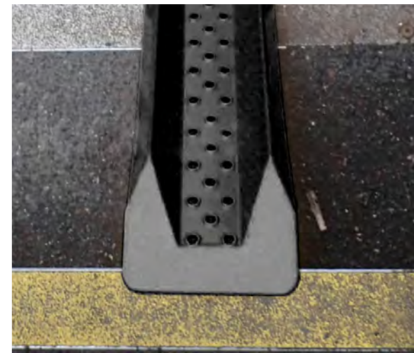
Top of Bike ramp for stairs
