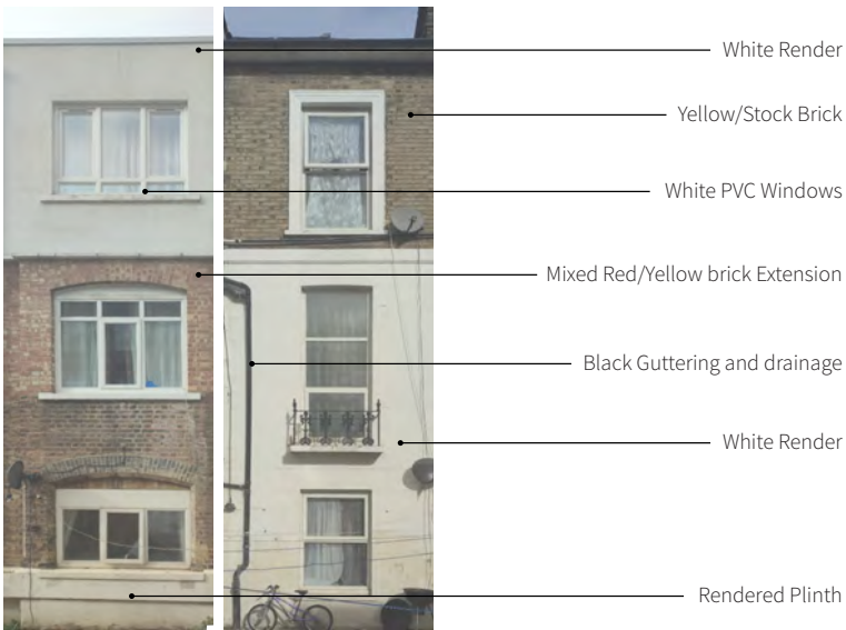
Existing rear extension & original building materials (respectively)
