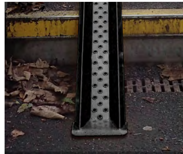
Bottom of Bike ramp for stairs
