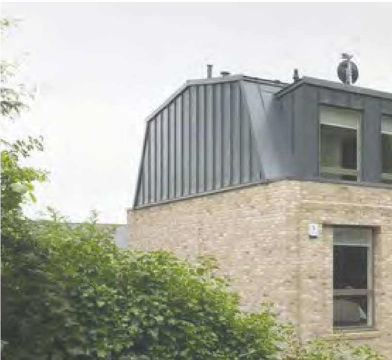
Zinc/Lead roof system example with standing seams
