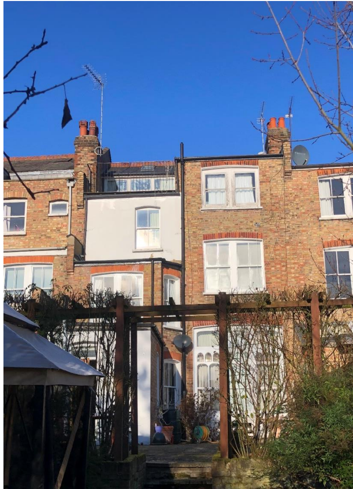
Fig.1 Rear View of No 49 The Avenue
