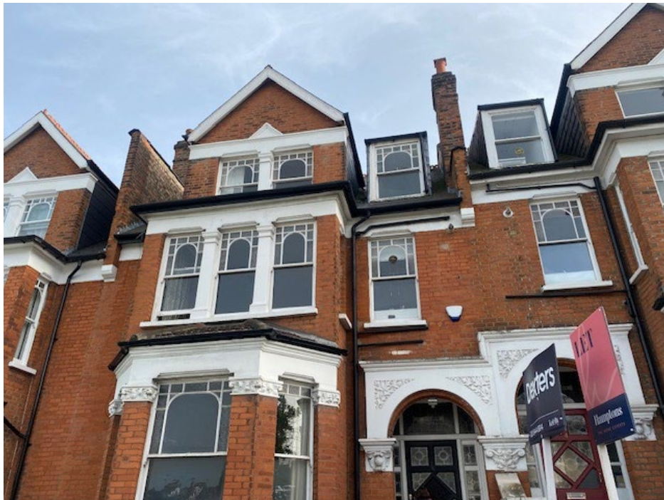
Fig.6 Front View of No 76
