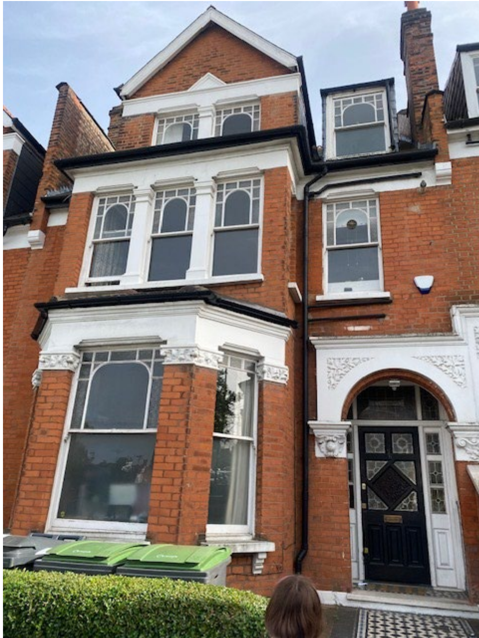
Fig.4 Front View of No 76
