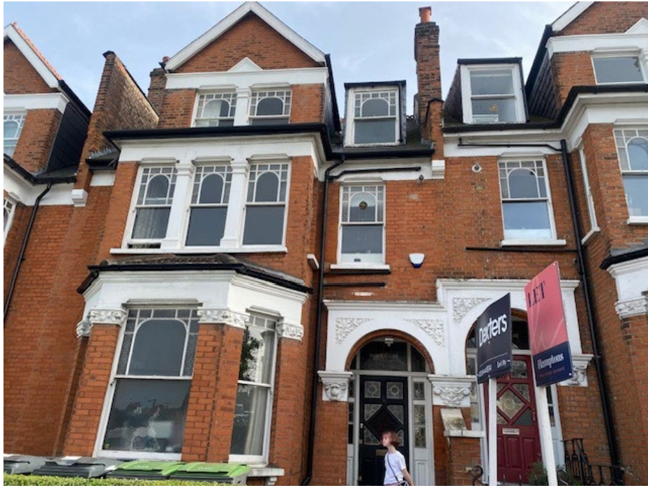
Fig.5 Front View of No 76
