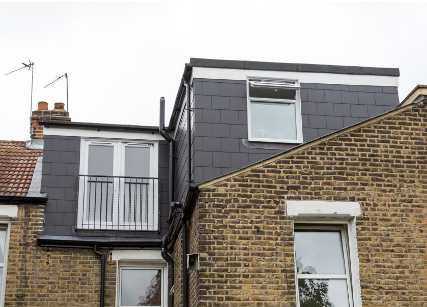
Existing Site Photograph_ Rendered Wall and Tile Hung Dormer Cladding
