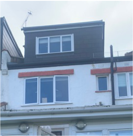
Existing Site Photograph_ Rendered Wall and Tile Hung Dormer Cladding
