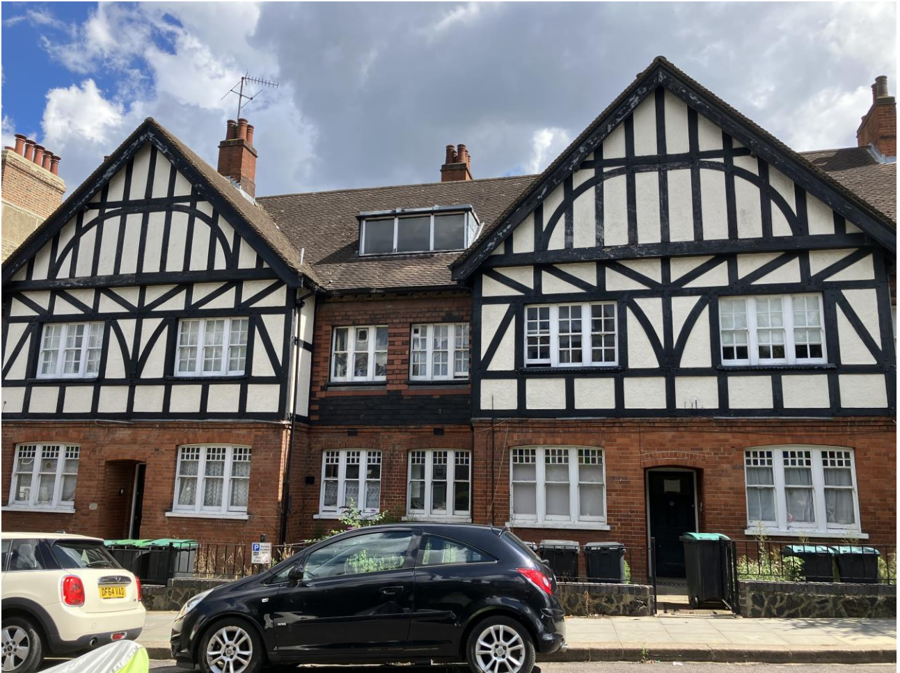
1-8 Firemen's Flats, Glebe Road, London, N8 7DD
