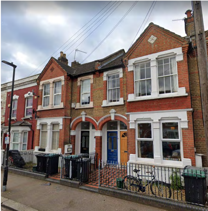
47 Grove Road East Elevation
