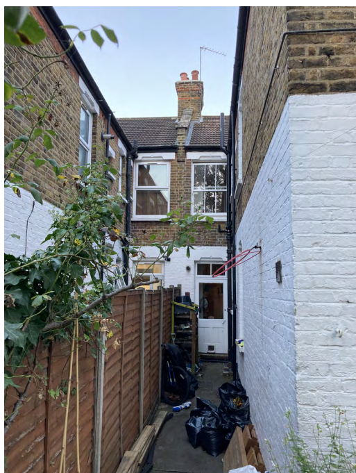
47 Grove Road West Elevation
