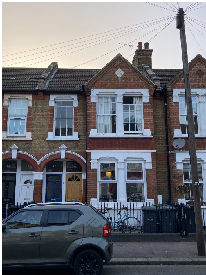
47 Grove Road East Elevation
