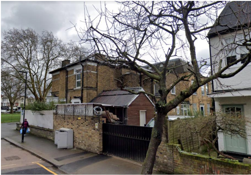
Figure 3: Rear elevation looking east along Lausanne Road
