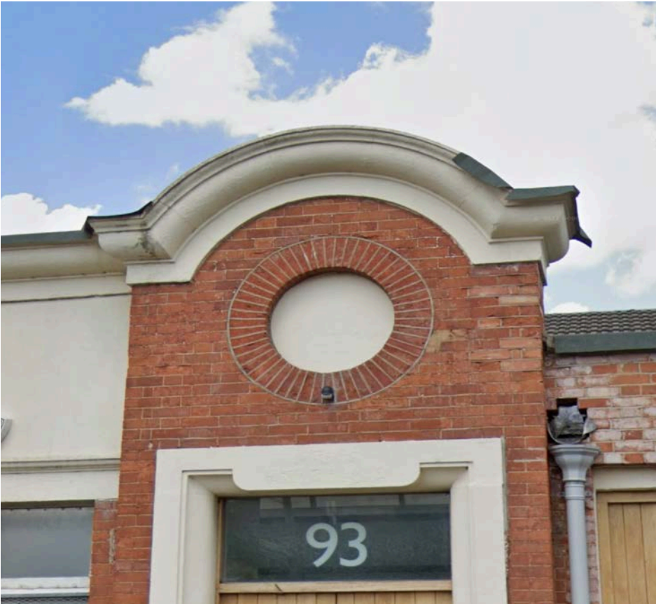
1 Facade Decoration - Vale Road
