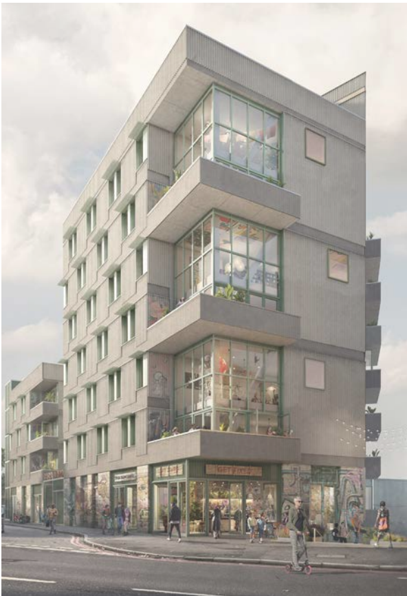
6 Misaligned Square Windows
